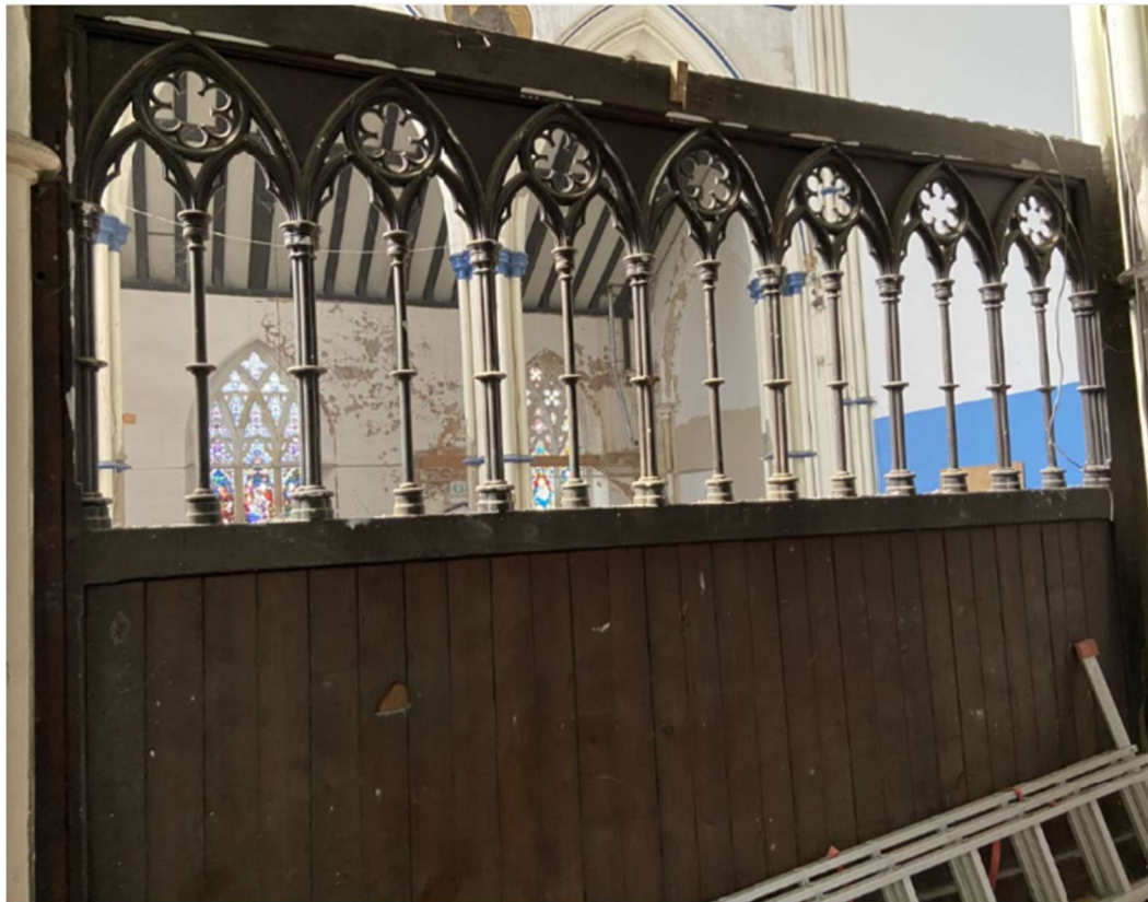
Fig 36 Existing timber rood screen
