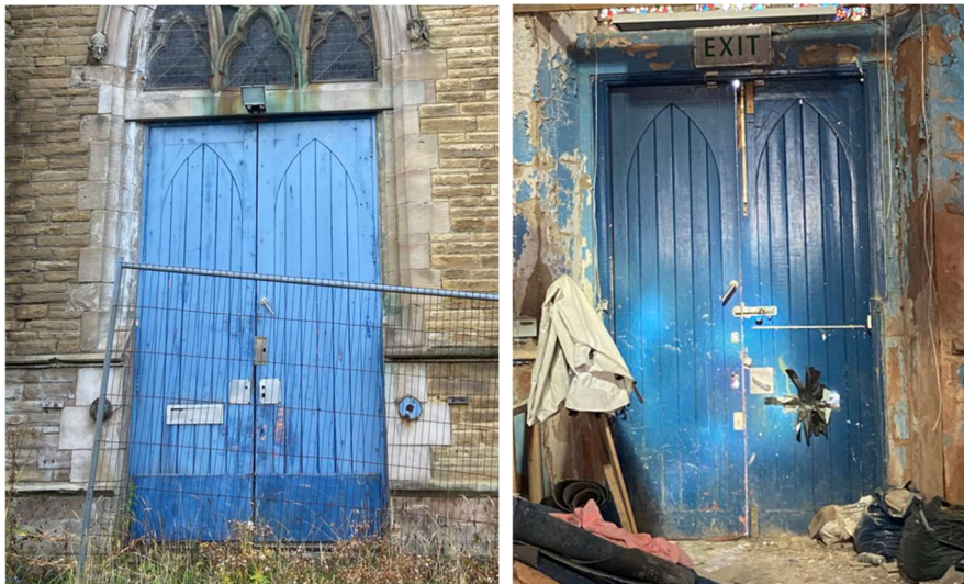
Fig 17 & 18 existing entrance door off St Marys Street
