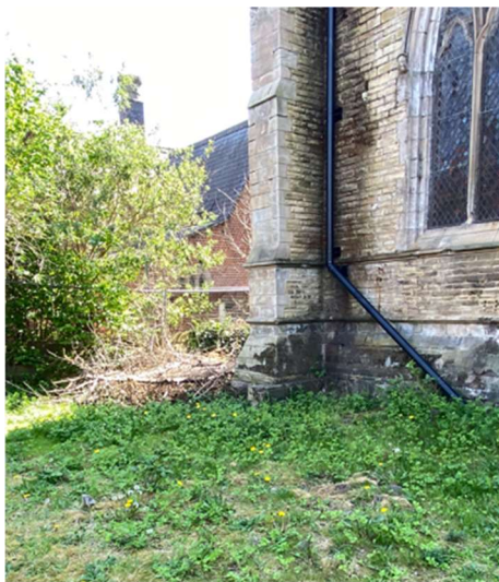
Fig 5 Temporary repair in upvc in 2024
