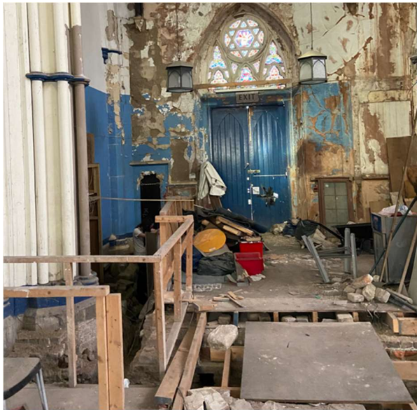
Fig 27 Raised timber floor added to main entrance doors
