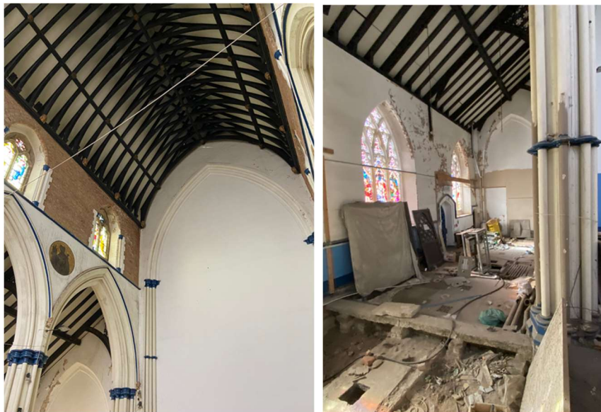
Fig 39 & 40 timber framed ceilings
