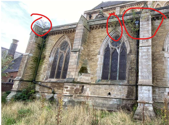
Fig 6&7 High level shrubbery within mortar joints
