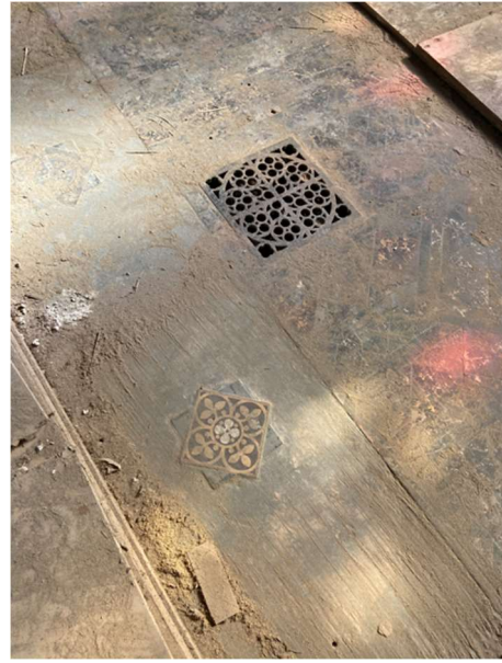
Fig 21 & 22 Encaustic tiles to former altar and inlaid to some steps and also showing metal grillage
