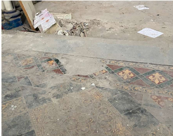
Fig 23 & 24 Infills to broken and missing tiles
