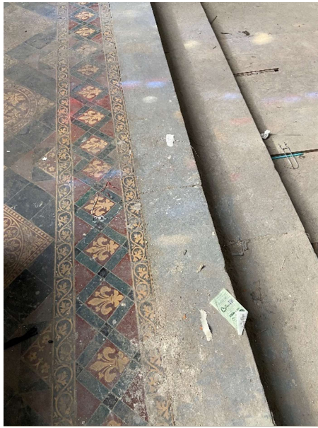
Fig 21 & 22 Encaustic tiles to former altar and inlaid to some steps and also showing metal grillage
