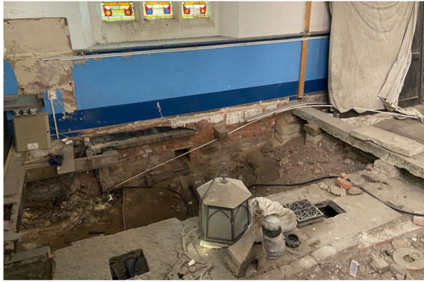
Fig 26 Areas where floors have entirely been removed, cast iron grilles retained
