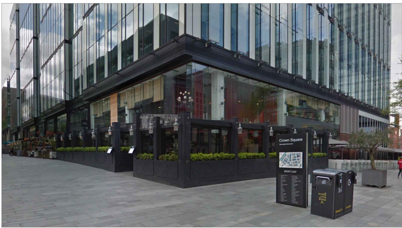
2017 Pergola from former restaurant Iberica
