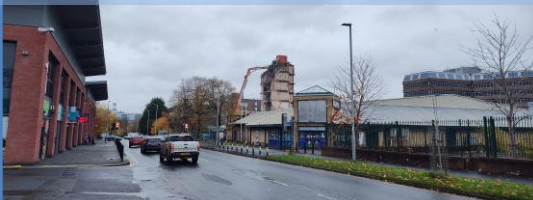
Approaching the site from the south on Rowlandsway
