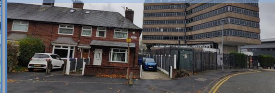
Separated by Wavell Road, family housing, offices and a data storage building occupy land to the east of the site
