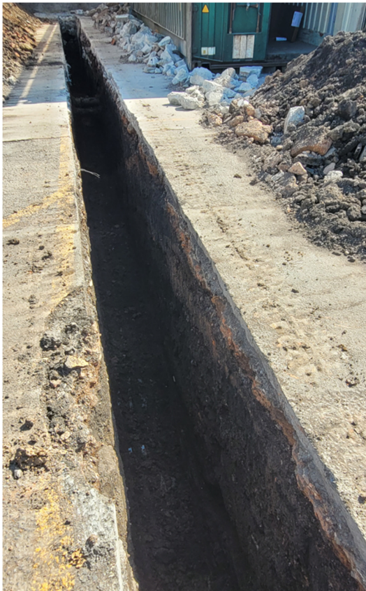
Photograph 1 – Trial Pit Viewing East
