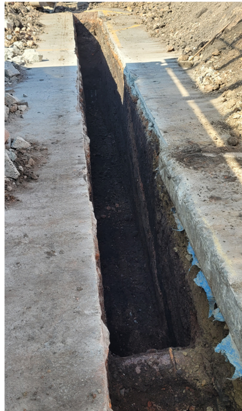
Photograph 2 – Trial Pit Viewing West
