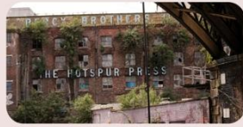
The Hotspur Press before the fire
