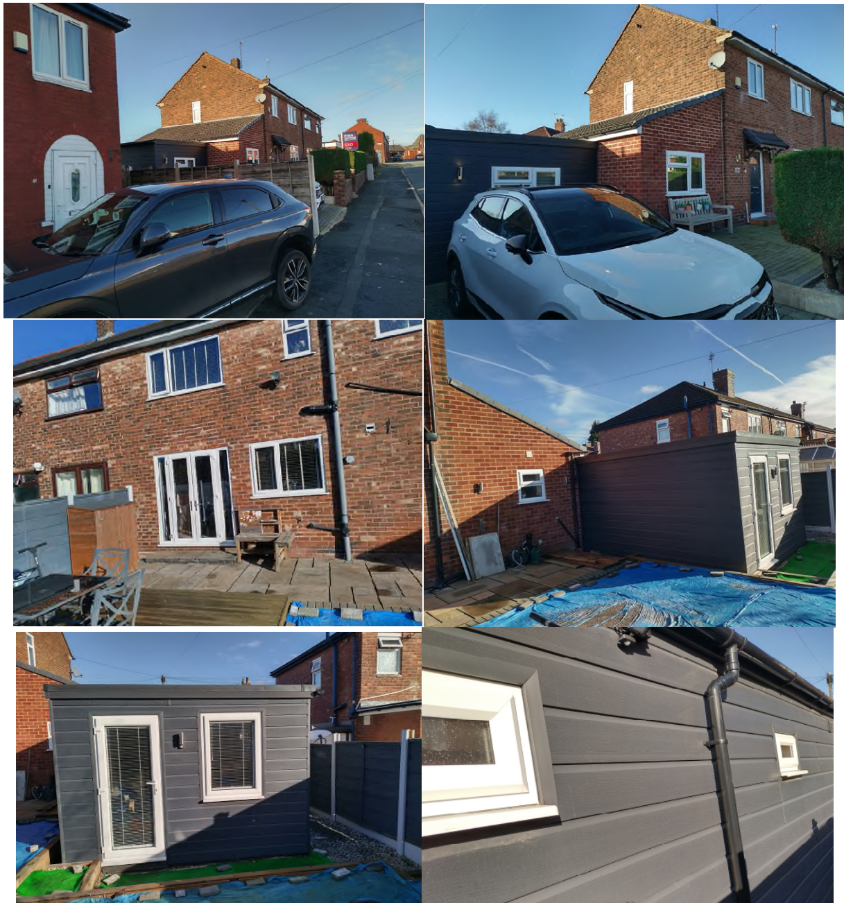
Fig.2 – Views of the front and rear of 44 Romney Street.
