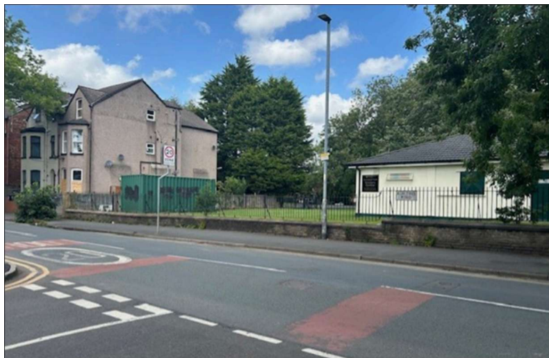
View of application site
