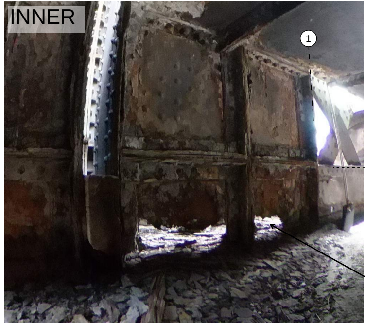
Holes to bottom of lower panels
