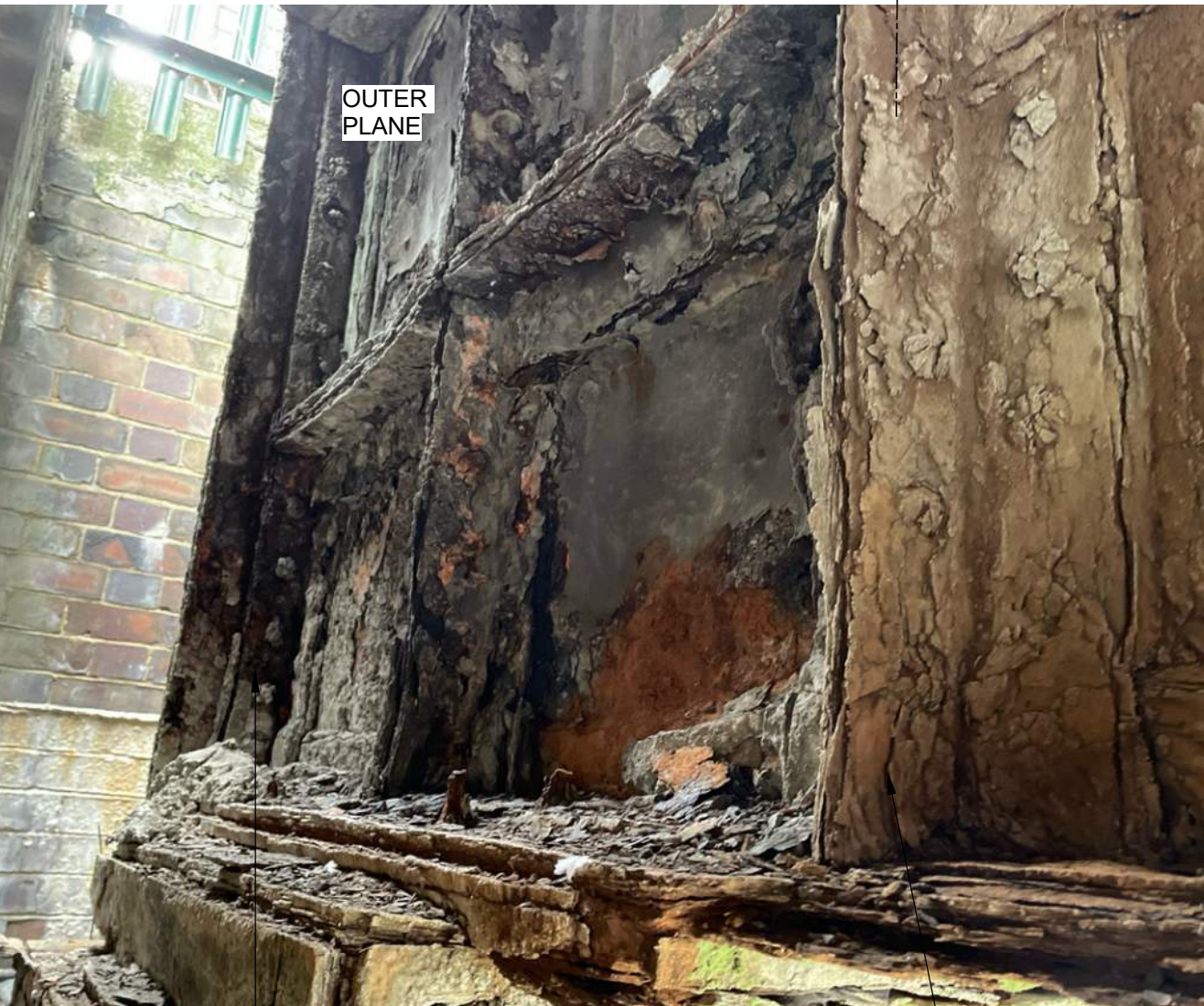
Span 8 North Elevation, Cornbrook End
