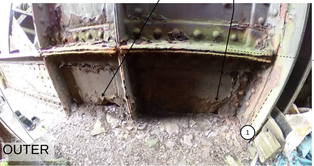
Holes to bottom of lower panels
