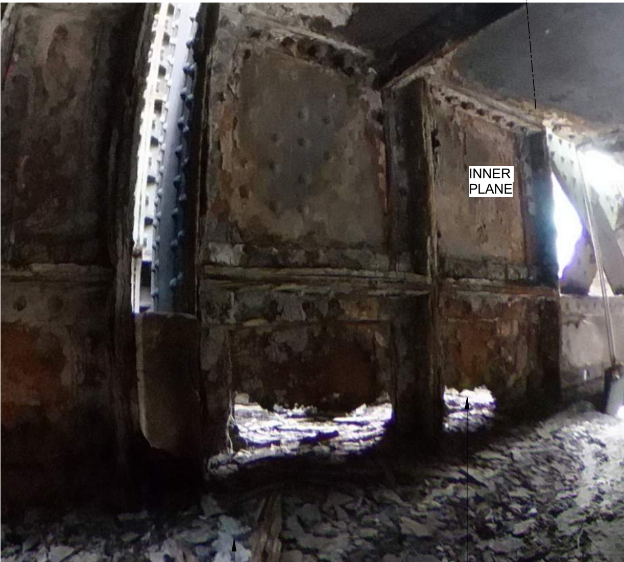
Span 7 North Elevation, Cornbrook End
