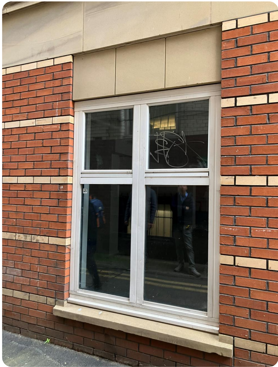
Existing Stone Lintel Fascia above Window
