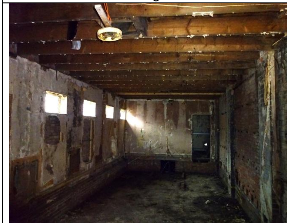
Area 1, GF1 interior – wooden floor and plasterboard ceiling removed
