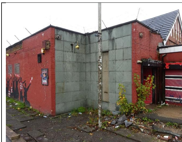
Area 1 to front of building – due for demolition
