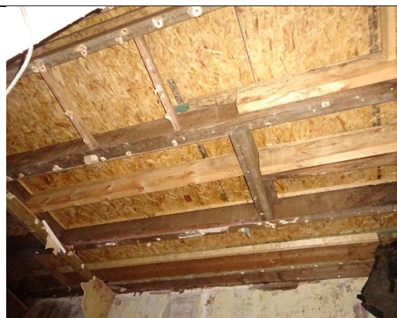
Area 1 – oriented strand board to flat roof
