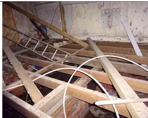
Area 1, GF2 interior – wooden floor removed revealing floor joists
