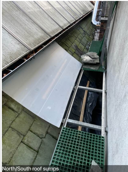
North/South roof sumps
