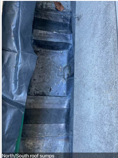
North/South roof sumps
