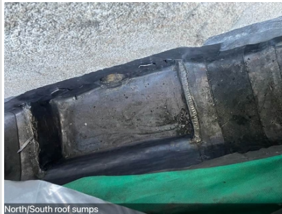
North/South roof sumps
