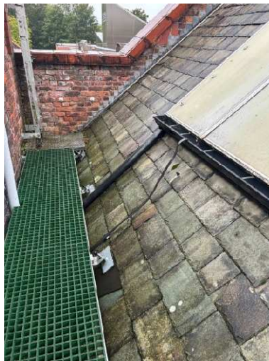
RW Gutter installed to discharge into existing gutter & hopper
