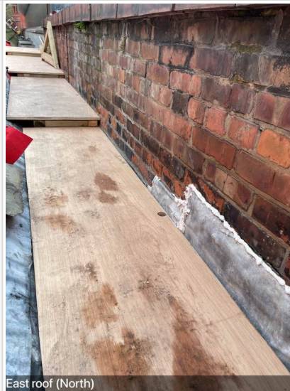
East roof (North)
