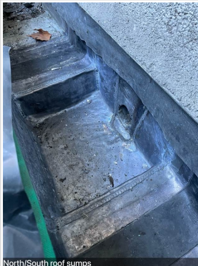
North/South roof sumps
