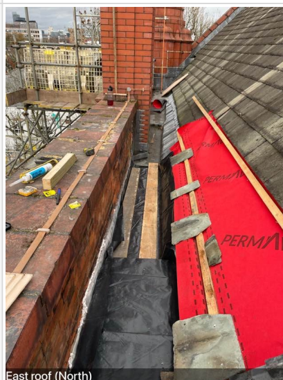
East roof (North)
