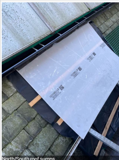
North/South roof sumps
