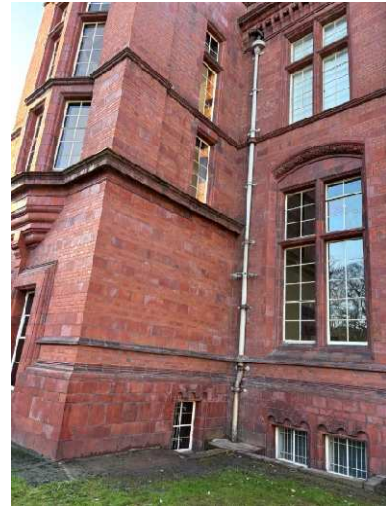
Existing view of hoppers & rwp
