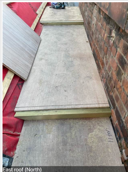
East roof (North)
