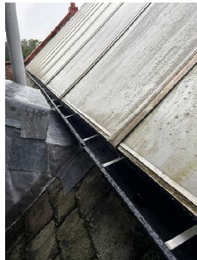
RW Gutter installed to discharge into existing gutter & hopper
