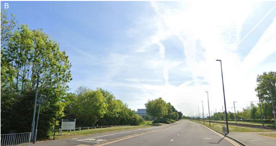
View from west Aviator Way
