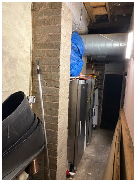
Image 2: Ground floor entry; Form linen store areas within recesses, with FD60SSC doors and frames, along with shelving internally. New FD60SSC door to Pub Kitchen.
