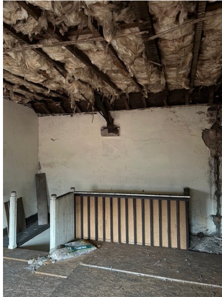
Image 5; New stair balustrades throughout to ensure compliance with height regulations and required strength. New fire rated stud walls to edge of stairs.
