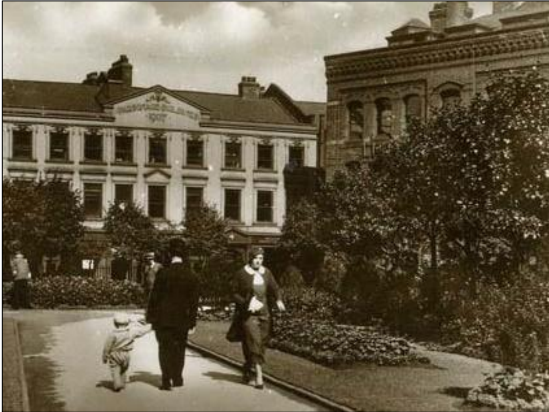
Figure 16. A view of Parsonage Gardens in the mid-1920s showing the dormers installed to the roof following alterations made by the Independent Order of the Rechabites.
