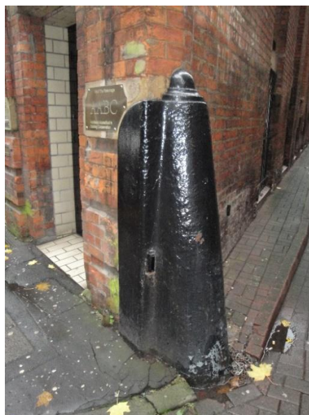
Figure 45: The original cast-iron corner bollard on the corner of Back College Land.
