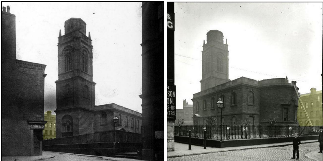
Figure 13. Two views of the west and east end of St. Mary's Church in 1891, in the process of demolition. The north elevation of the warehouse property facing North Parade can be seen (highlighted) enclosing the church.
