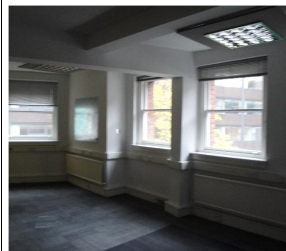
Figure 32: The attic third floor showing original sash windows.
