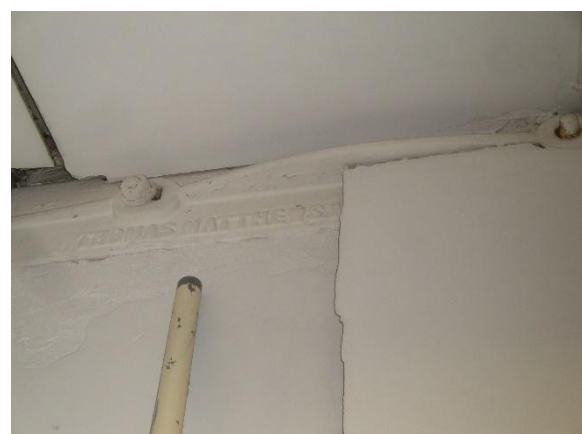
Figure 39: A structural cast-iron brace to the ceiling structure on the ground floor on No. 2, showing the makers mark.
