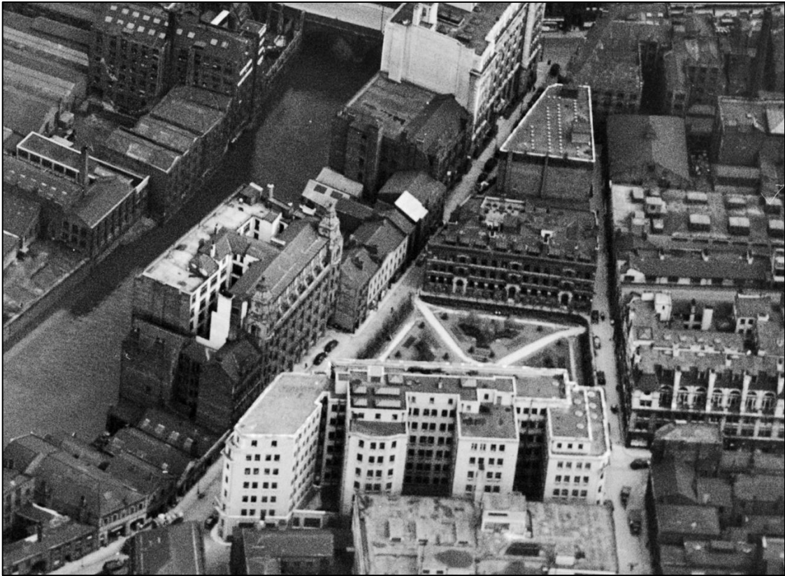
Figure 17a. Aerial view of Parsonage Gardens and the One North Parade site in 1938, a year before the construction of the new store at Kendal Milne to the south, showing how the gardens and buildings were tightly enclosed at that time. All sides of the gardens featured and was fronted by built form of differing height, mass and scale.
