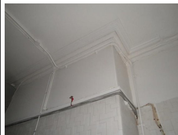
Figure 38: A small section of original plaster cornice around the blocked chimney breast on the ground floor of No. 2.
