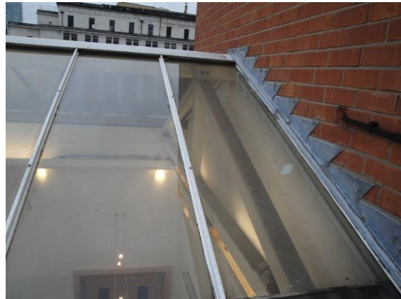
Figure 35: The modern light well roof and structure.
