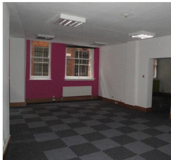
Figure 28: The ground floor office floor looking out onto Back College Land, showing the original sash windows and modern suspended ceiling, carpet and skirtings.
