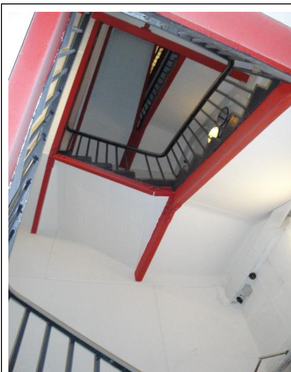
Figure 30: The inserted modern fire escape to the rear of the building, dating to the 1980s/1990s. This staircase cuts through every floor of the building.
