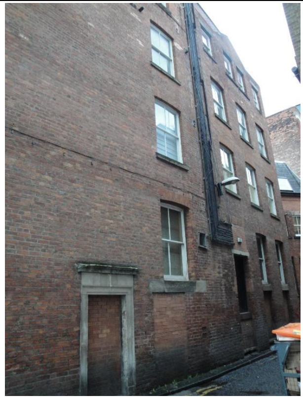
Figure 21: The eastern elevation along College Land, showing the utilitarian appearance and former loading bays.
