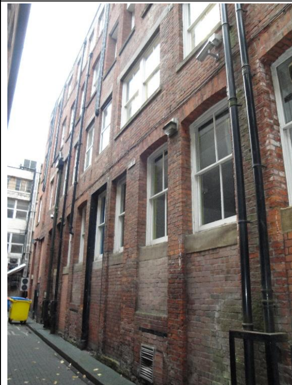
Figure 22: View from St Mary's Parsonage into Back College Land, showing the many former hoist openings to the ground and first floors.
