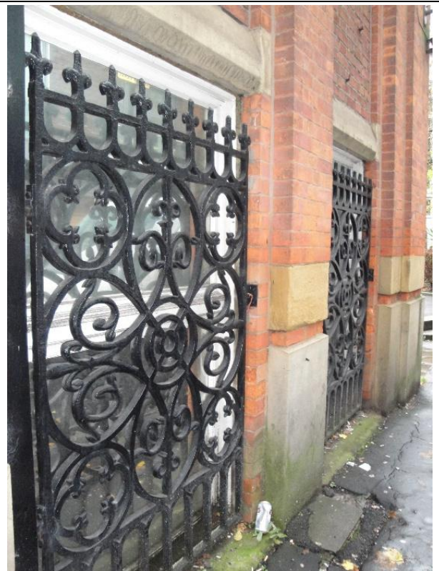
Figure 23: The remaining cast-iron basement window grills on the St Mary's Parsonage elevation.
