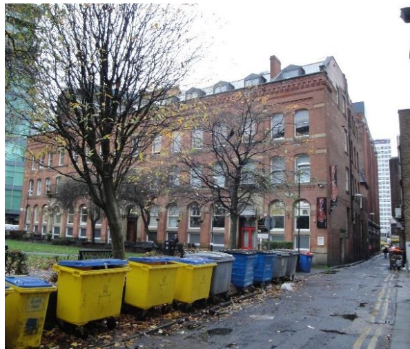
Figure 18: The north elevation on North Parade (2019)
