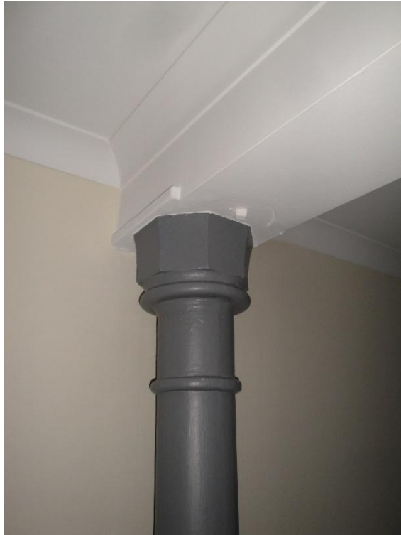
Figure 50: One of the many exposed original cast-iron column capitals, and modern cornice.
