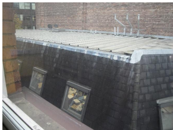
Figure 44: The modern roof structure, coverings and roof lights of No.5 Parsonage. .
