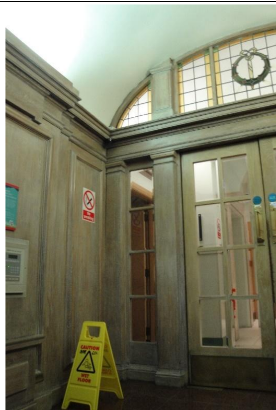
Figure 25: The c1920s internal panelled vestibule and glazed screen.
