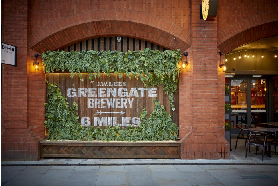
Image 1 – Existing reclaimed timber external store enclosure wall will be removed as part of the proposed works and will be replaced with new powder coated aluminium glazed screen in colour to match Founders Hall existing doors and screens. The existing reclaimed timber planter in front of the enclosure wall will be retained.
