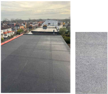
Concrete flat roof with bituminous felt covering
