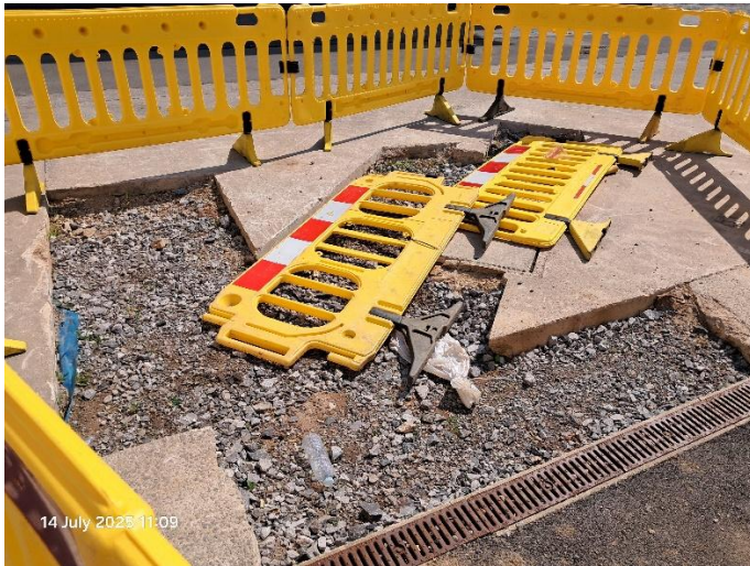
13. Facing east. Close up of united utilities works.
