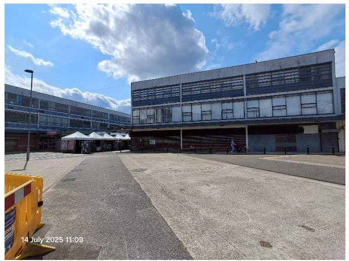
14. Facing southeast, view across concrete hardstanding towards main buildings.
