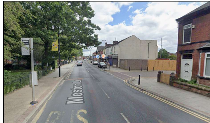
Plate TS6 - Moston Lane looking East at Ebsworth Street Junction (Note eastbound bus stop)
