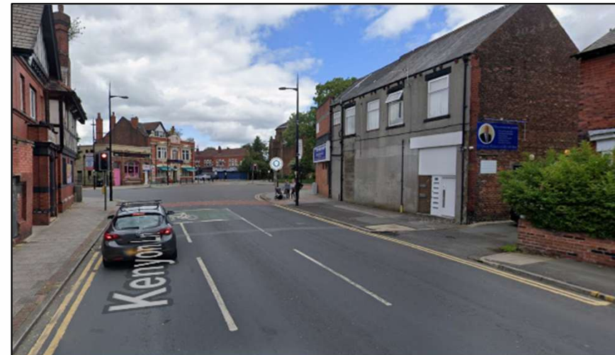
Plate TS10 - Kenyon Lane Approach to Moston Lane Junction
