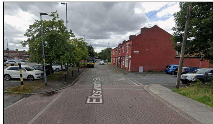
Plate TS2 - Ebsworth Street Frontage to Car Park (looking South)
