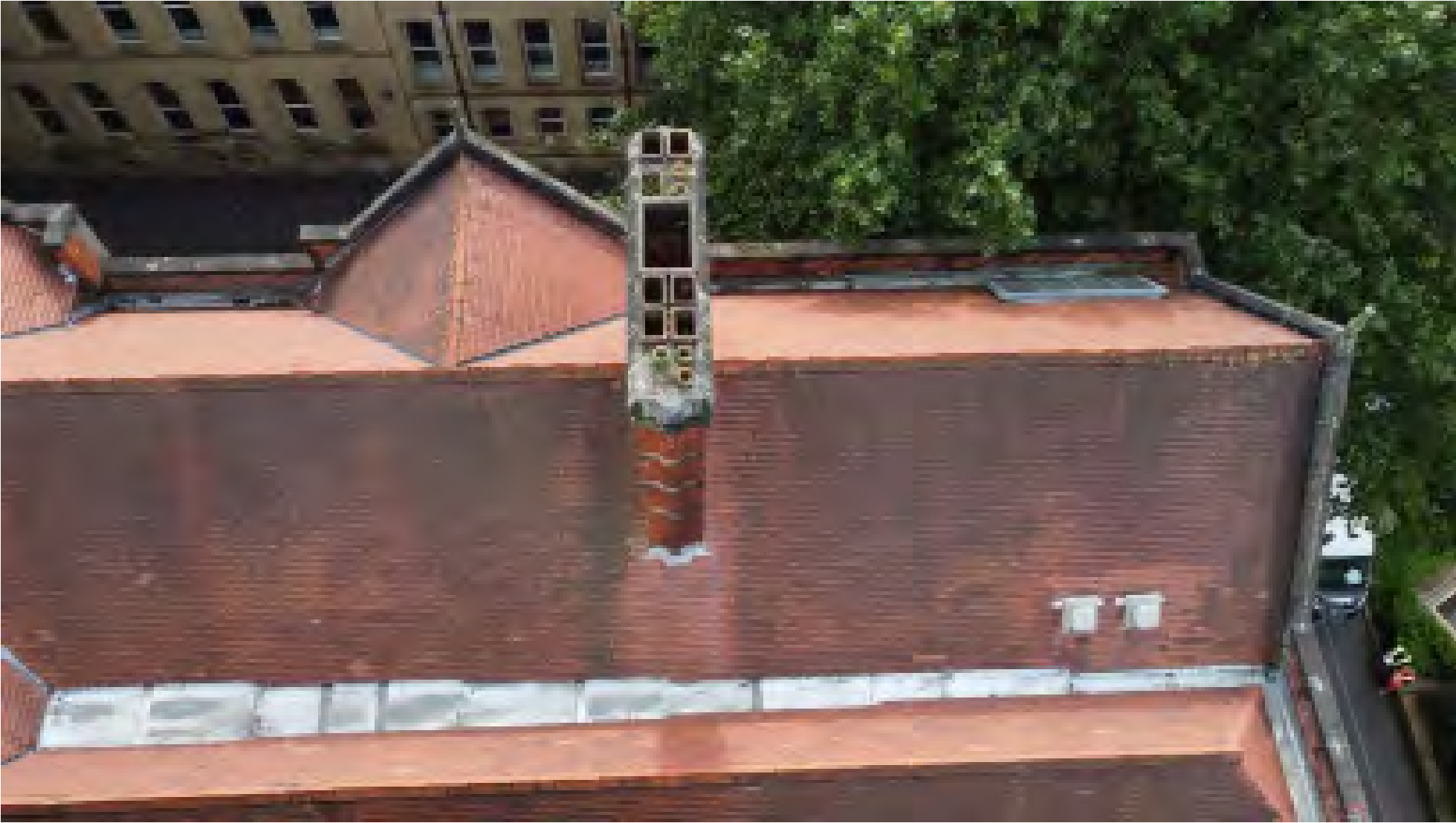
▲ Existing Lead Gutter over Corridor
