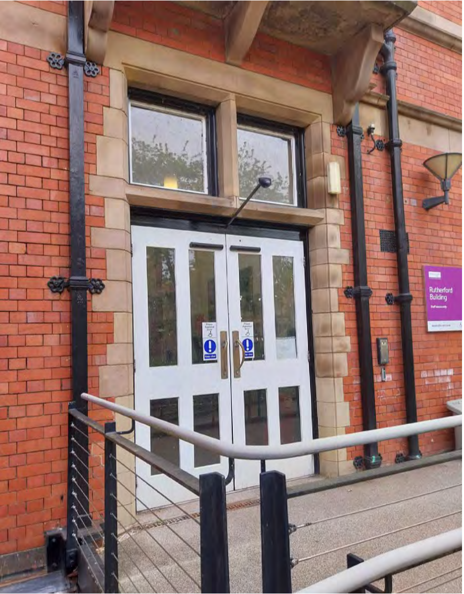
▲ Replacement of Entrance Doors to West Elevation
