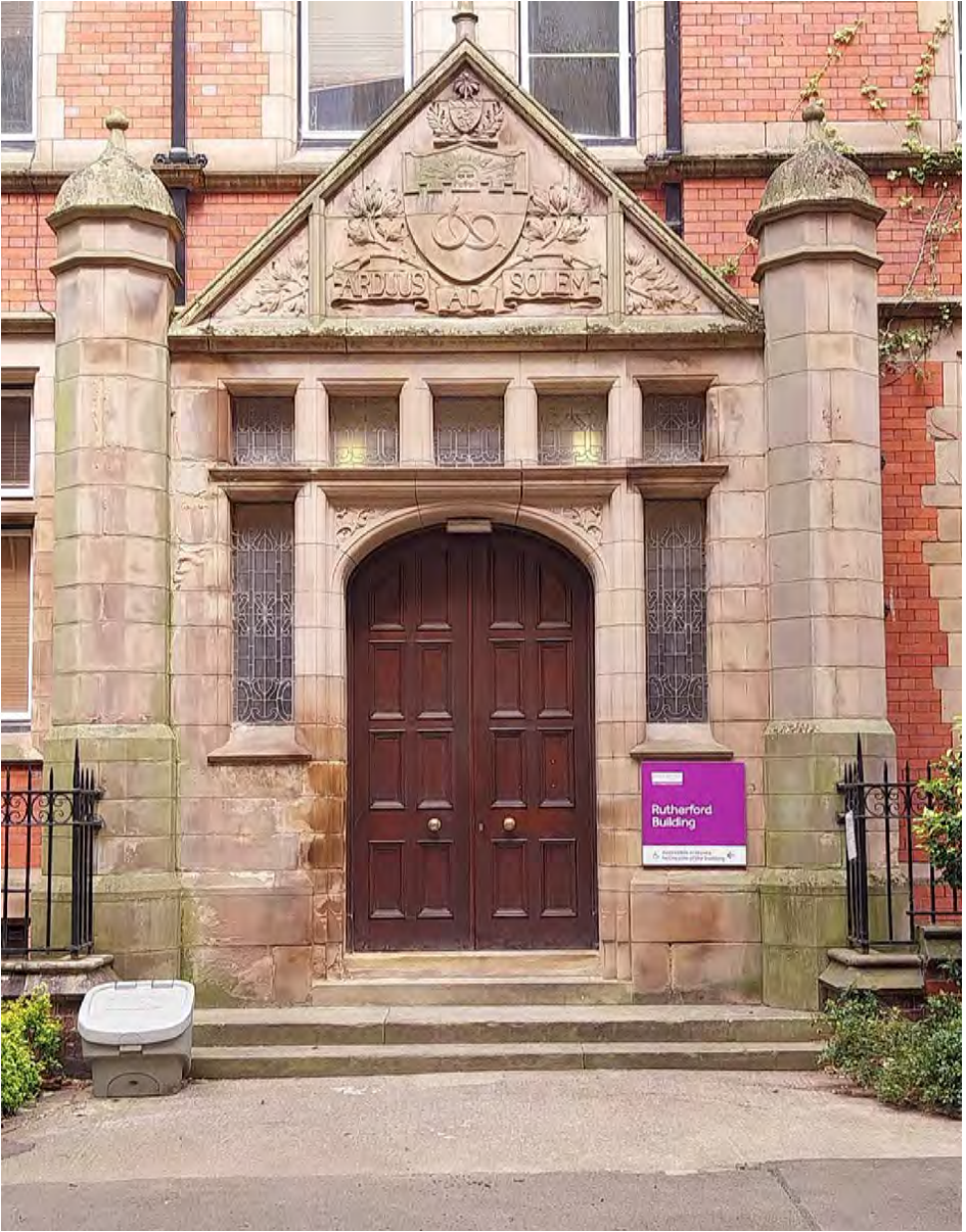
▲ Stonework + Leadwork Repairs to Main Entrance on Coupland Street
