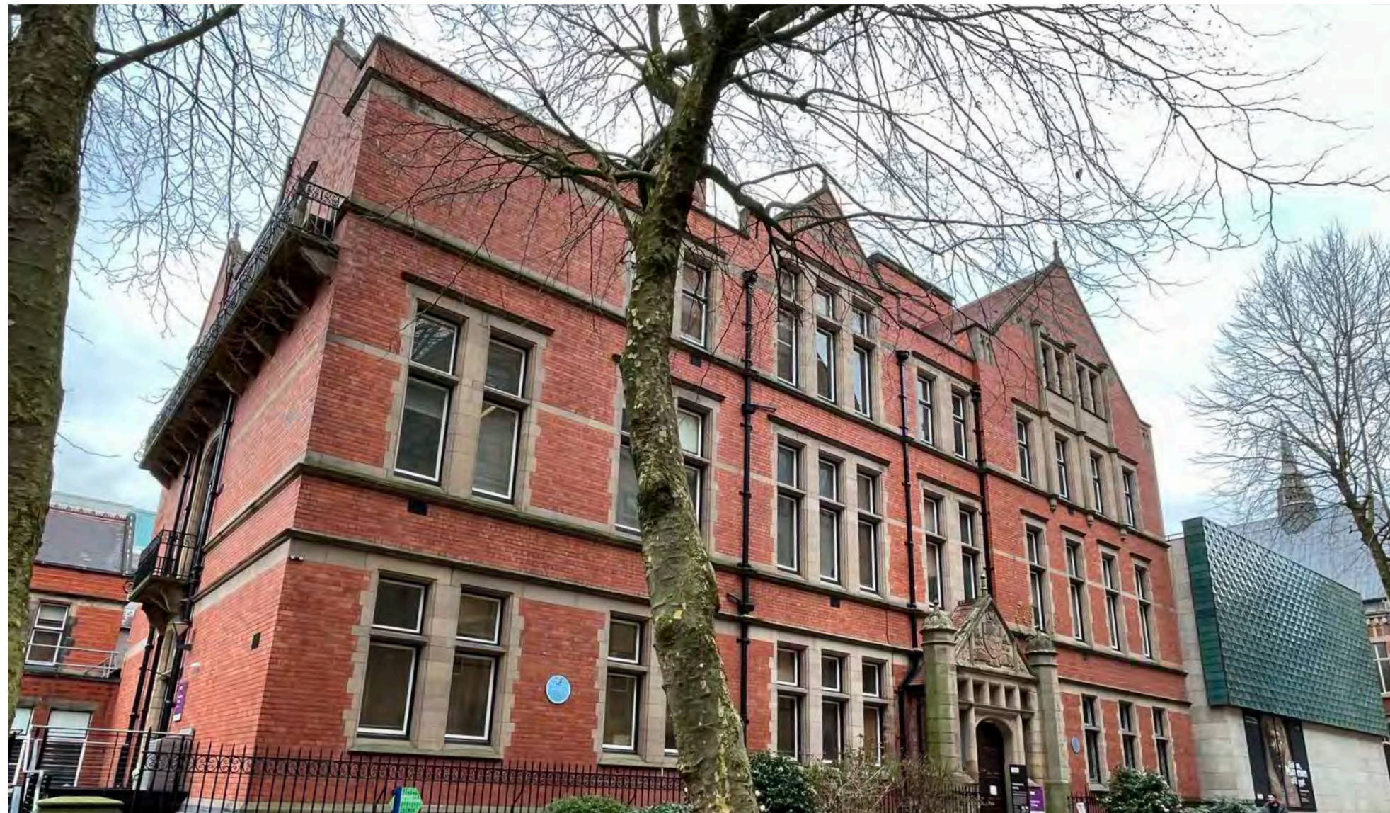
▲ Coupland Street External Facade
