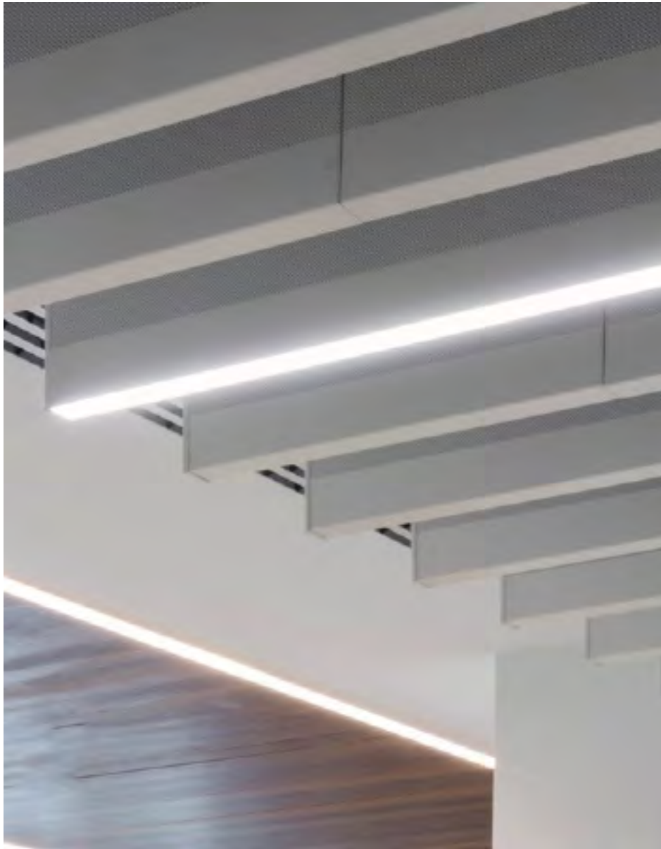
▲ Integrated Lighting with Linear Acoustic Baffles
