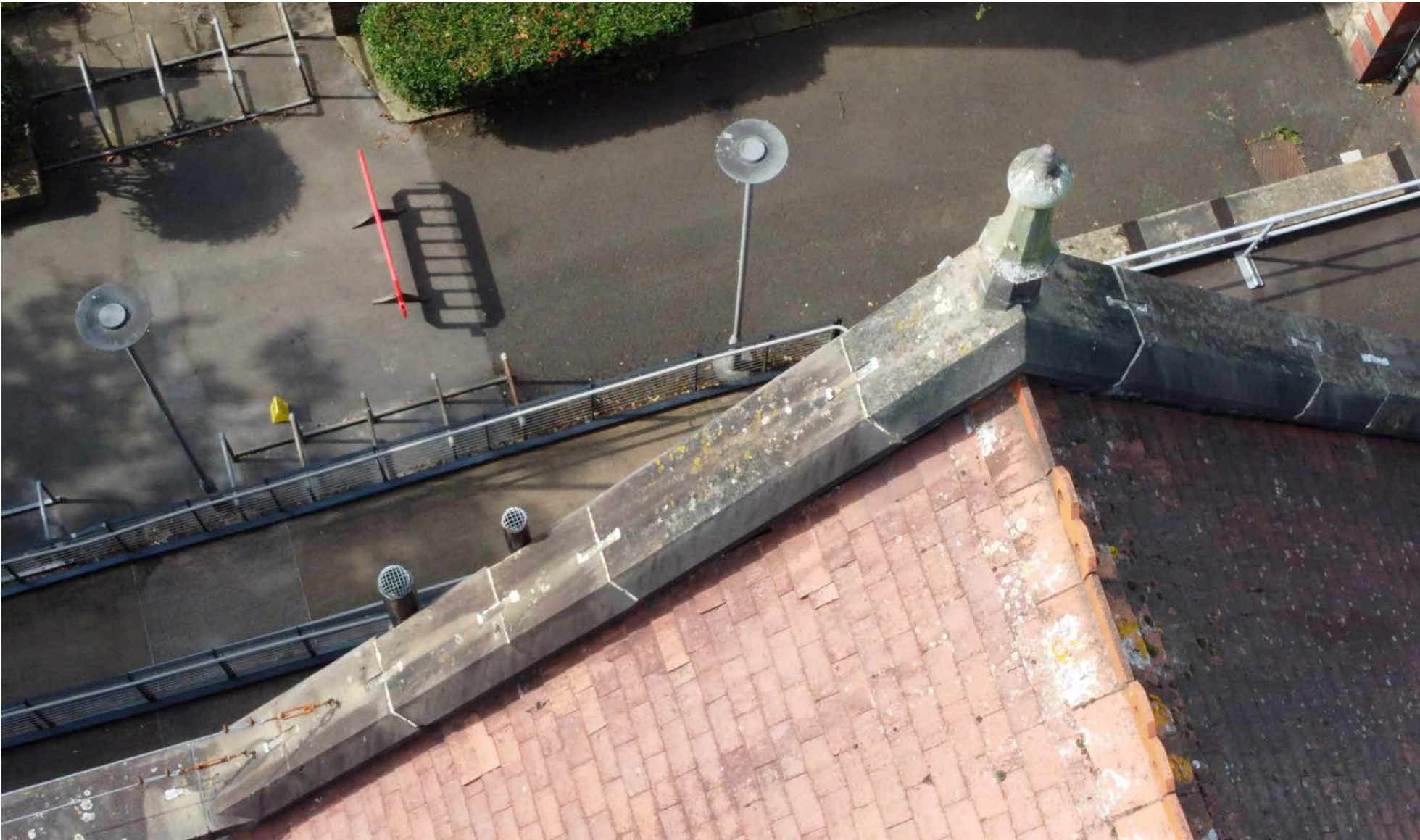
▲ View of Roof
