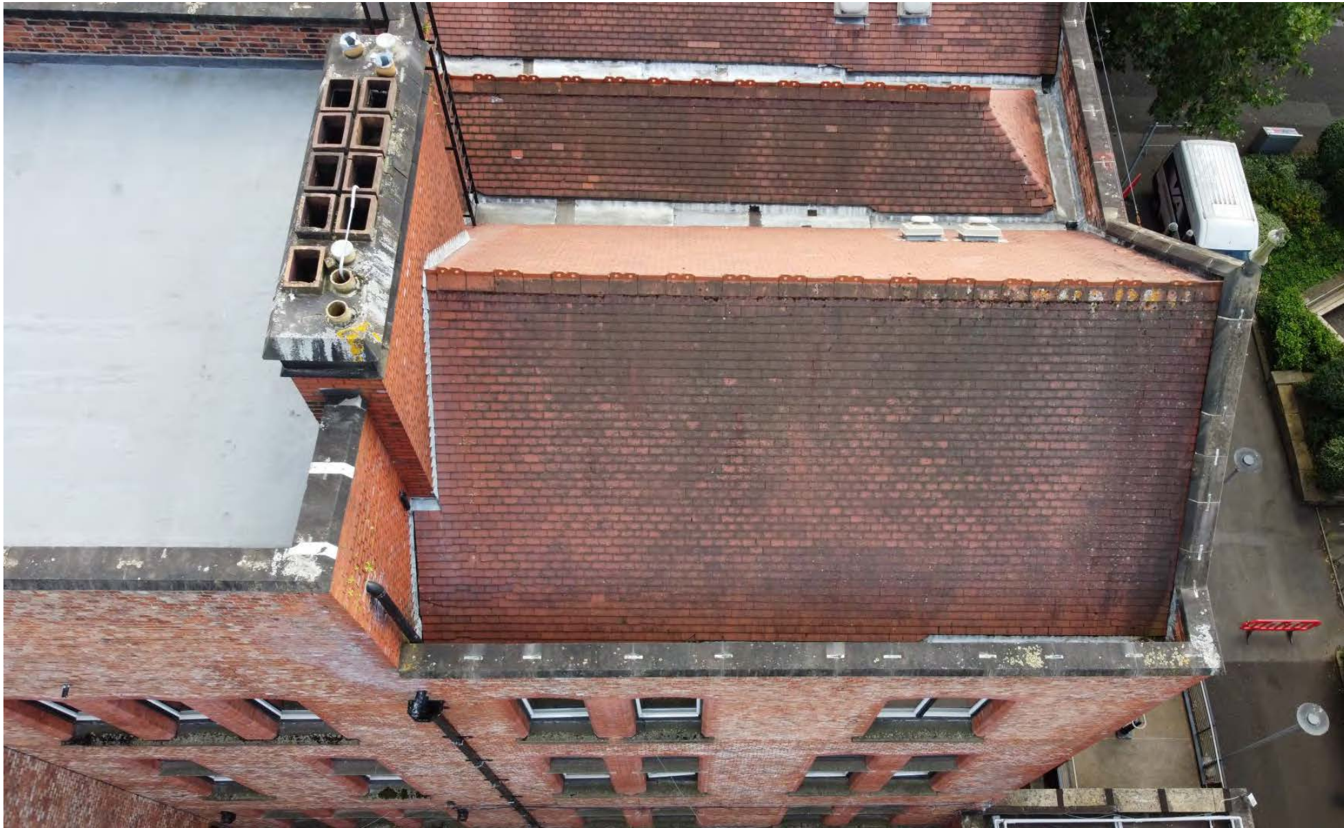
▲ View of Gable Roof, Chimney Breast and Flat Roof
