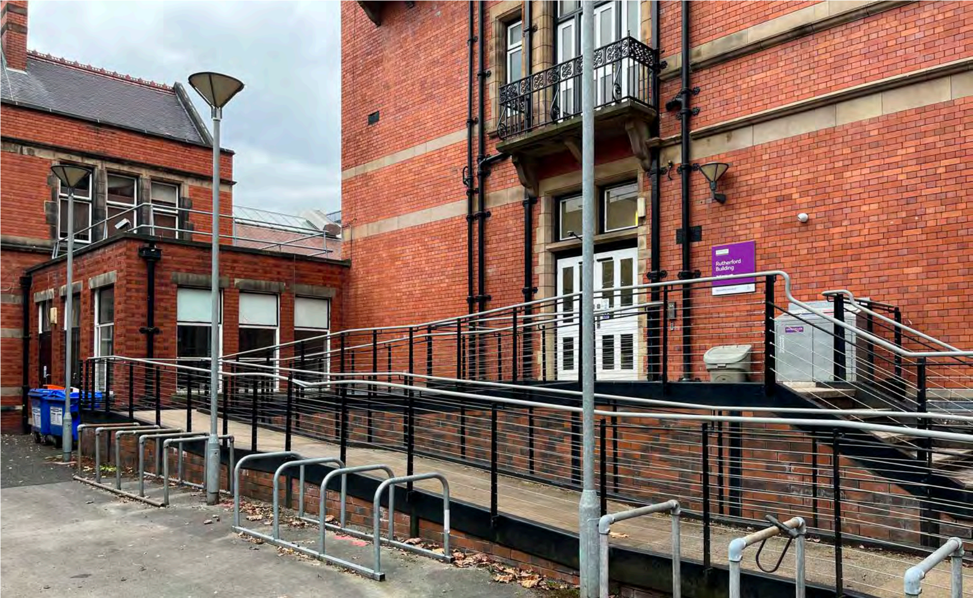
▲ Remodelling and Upgrade of 1990's Access Ramp and Stairs to the West Elevation
