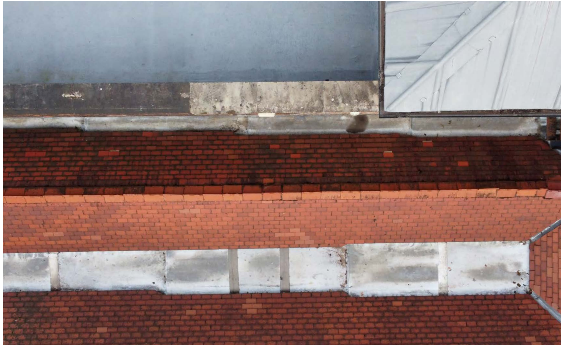
▲ View of Roof from Drone
