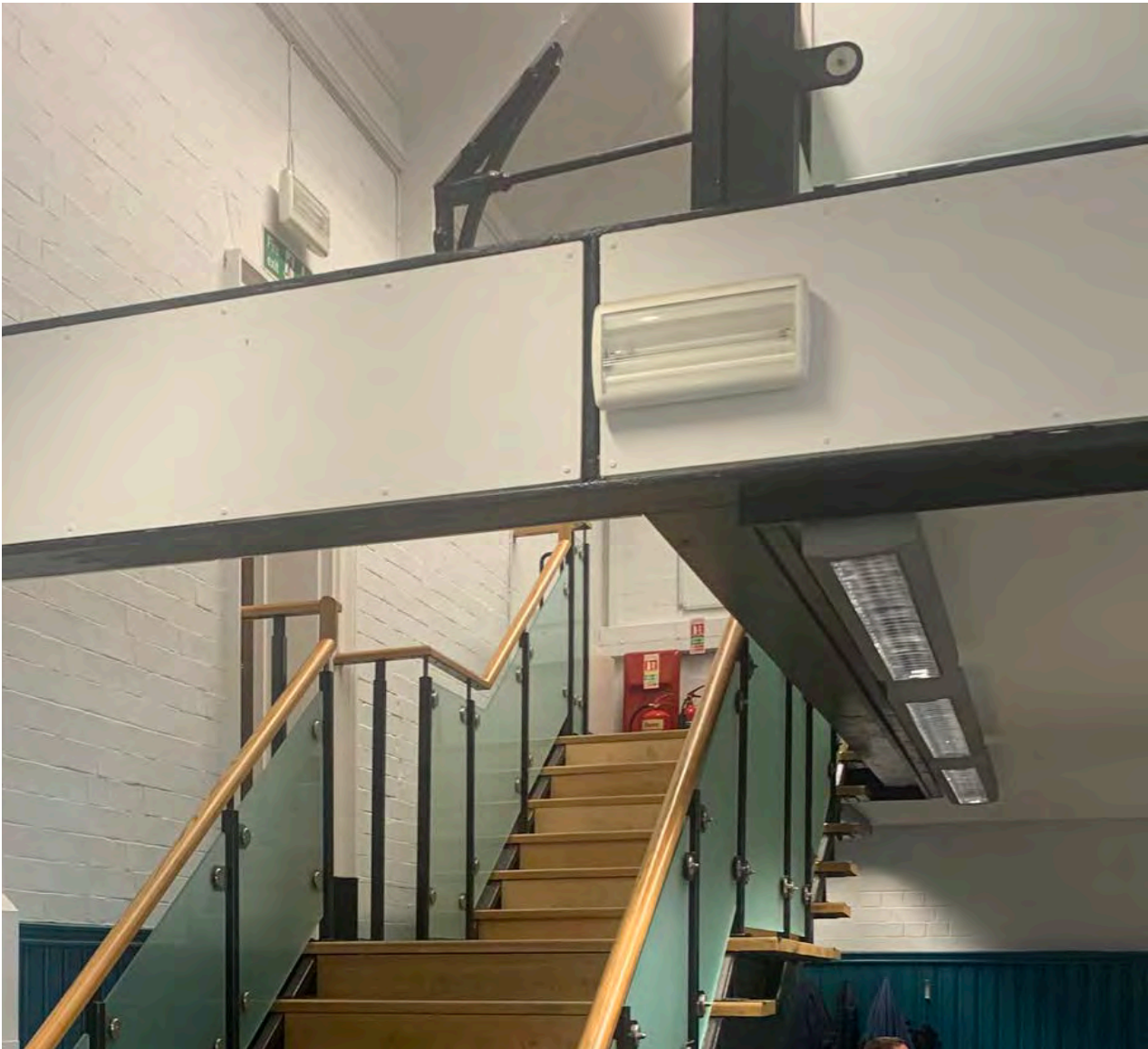
▲ Cladding Added to Mezzanine Floor Fascia in 1990s to be removed
