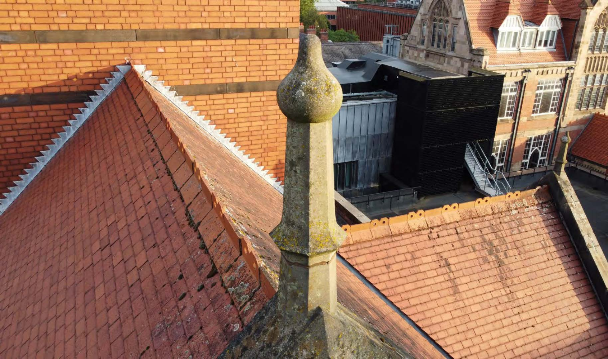
▲ View of Roof from Drone
