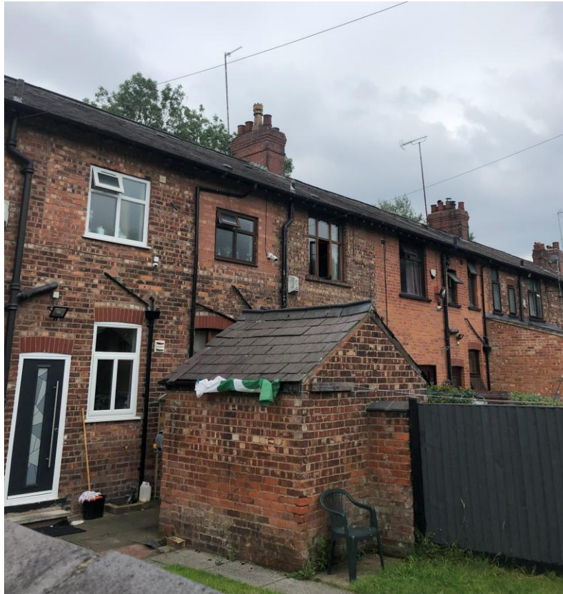
Figure 17. Existing relationship between the applicant property and no.91 Hazelbottom Road with existing outhouse
