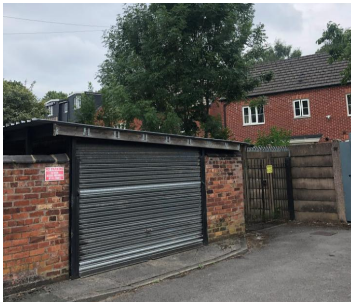
Figure 7. View of roller shutter within boundary wall to be removed as a result of the proposal
