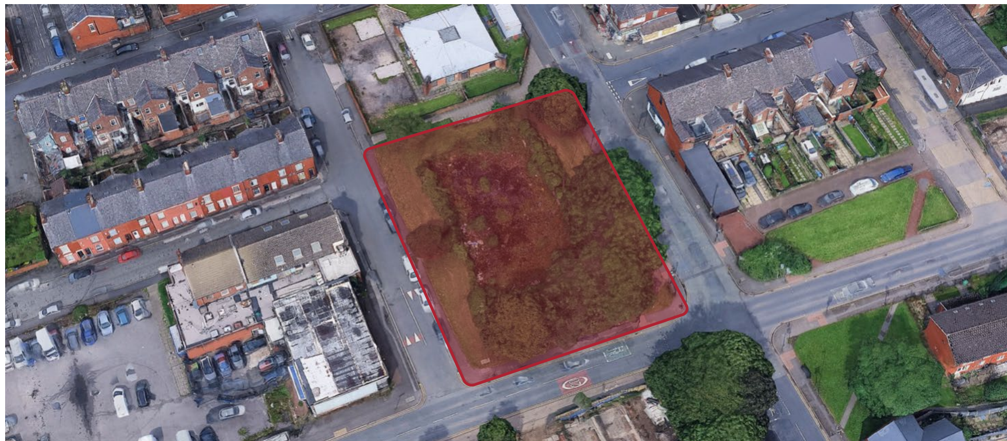
Image 2 - Existing Site 3D-aerial view
