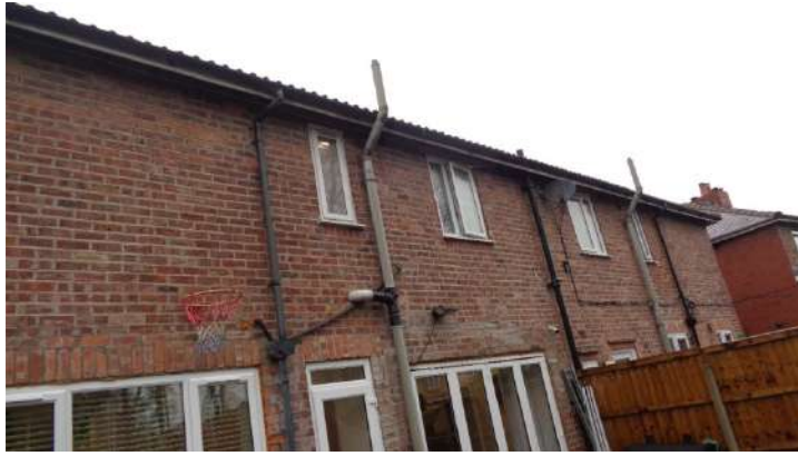
Rear of Application Property.
