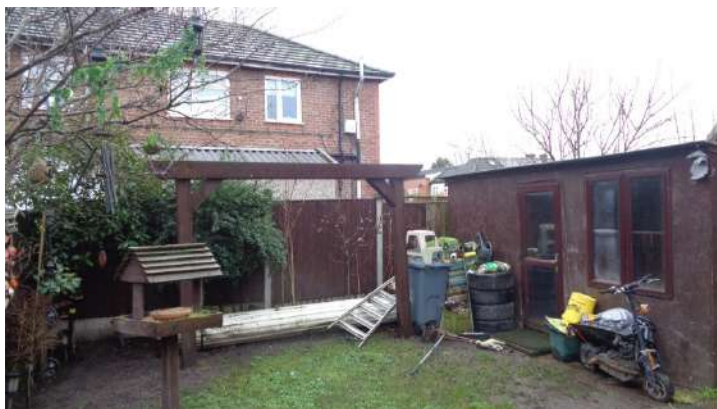
Rear of Application Property.
