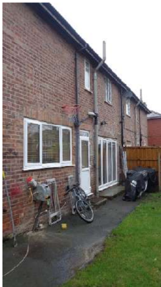
Rear of Application Property.
