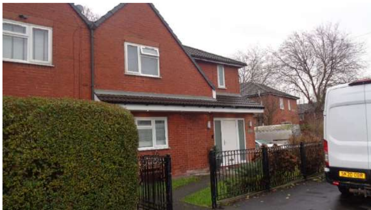
Front Elevation to Application Property.
