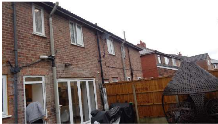
Rear of Application Property.
