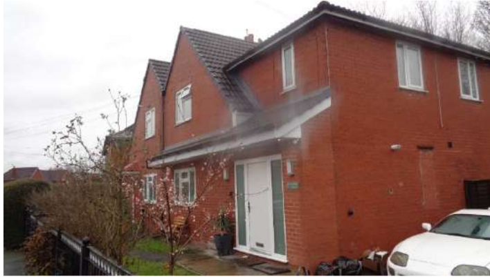
Front Elevation to Application Property.
