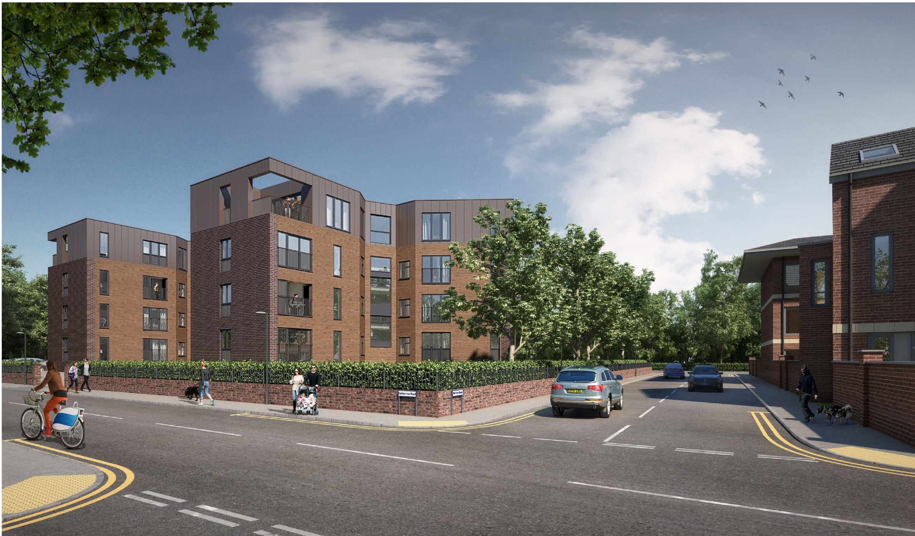
BERKELEY COURT, 150 BURY OLD ROAD MAY 2016
