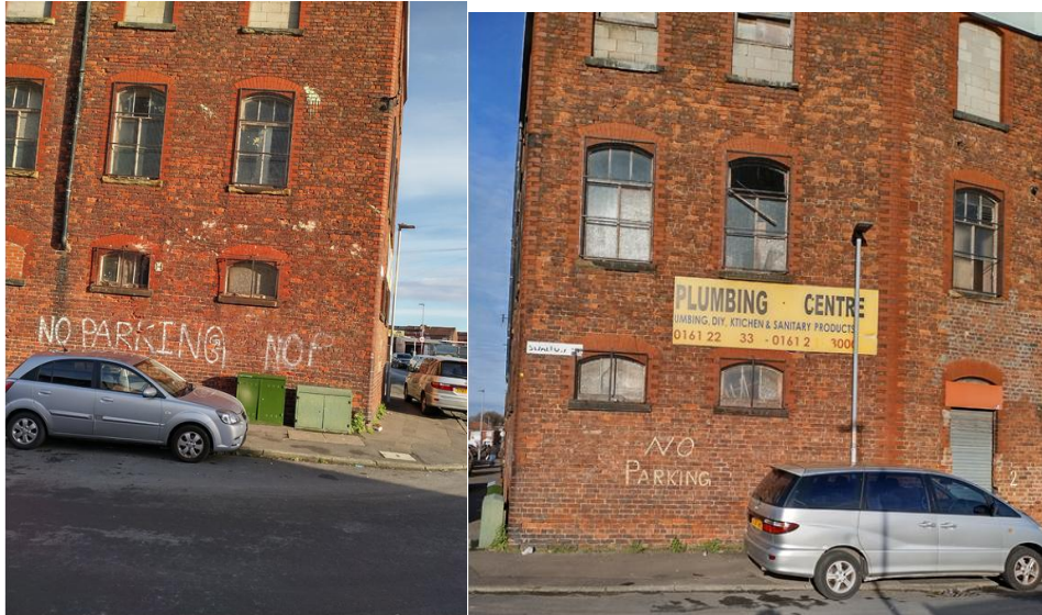
Fig.2 – Views of the application site
