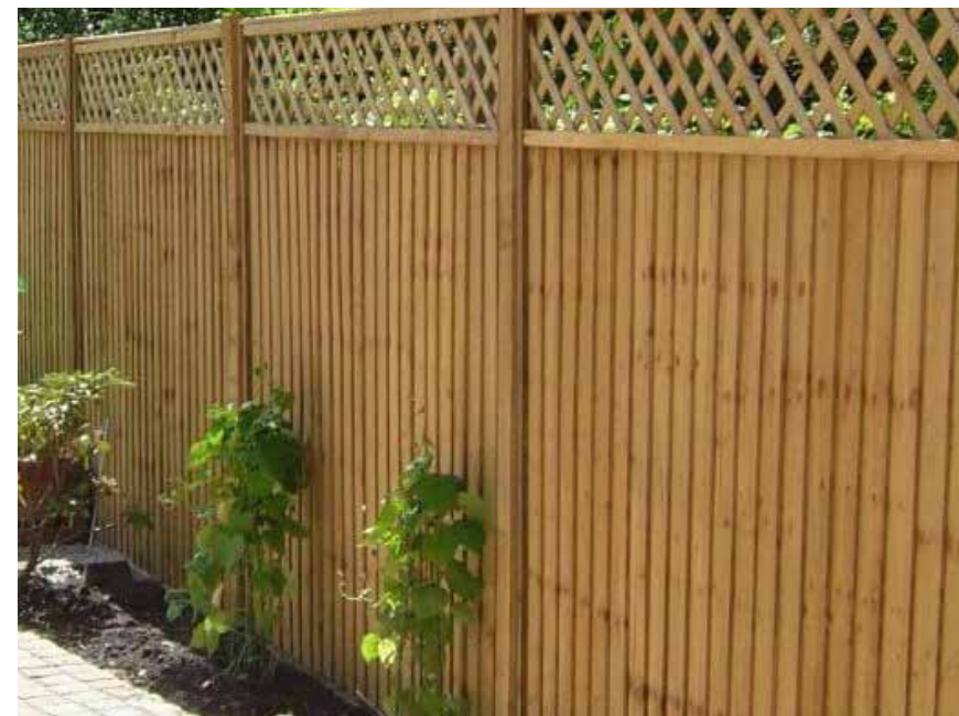
New 2.4m high boundary - tongue and groove fence with 0.3m high trellis
