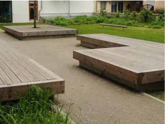
Reconstituted timber decking platforms for informal play and seating
