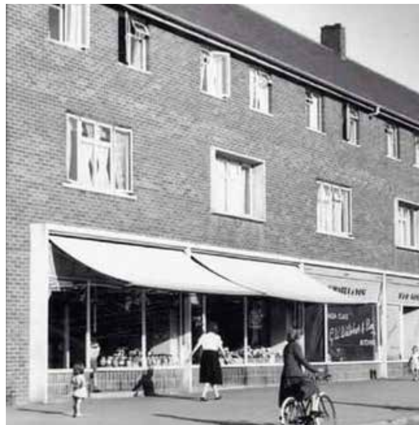
White base with canopies and glazed bricks to retail units
