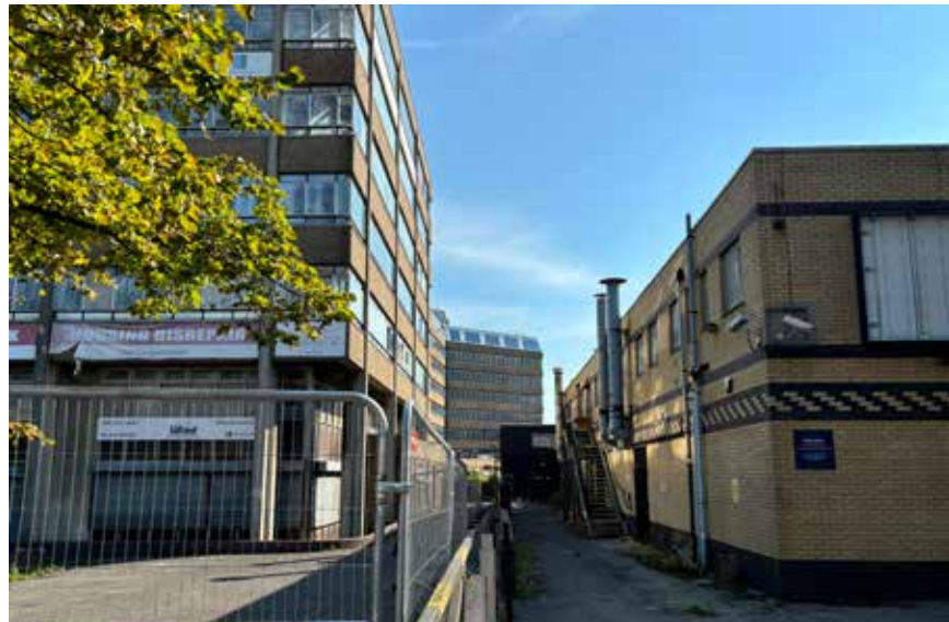
Photo B - view east of site boundary between existing Alpha House (left) and Bingo hall (right)
