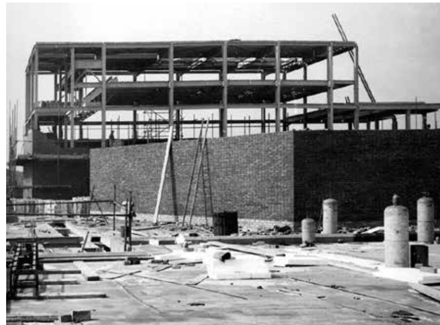
Modern construction methods were used for the new Civic Centre
