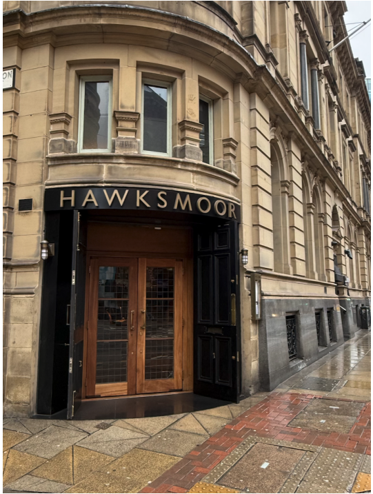
EXISTING ENTRANCE AT HAWKSMOOR, DEANSGATE
