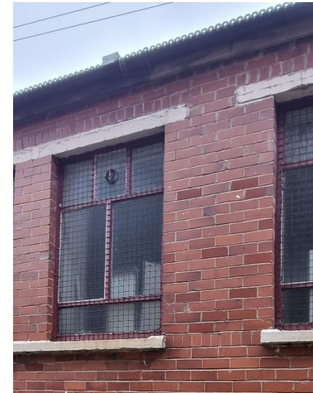
Typical existing window to be replaced
