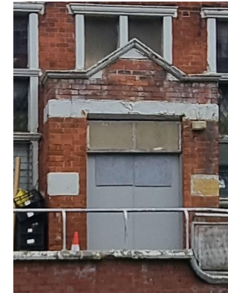
Existing entrance door to building (b) to be replaced
