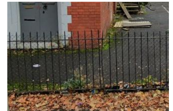
Existing metal railings on site, assumed to be original
