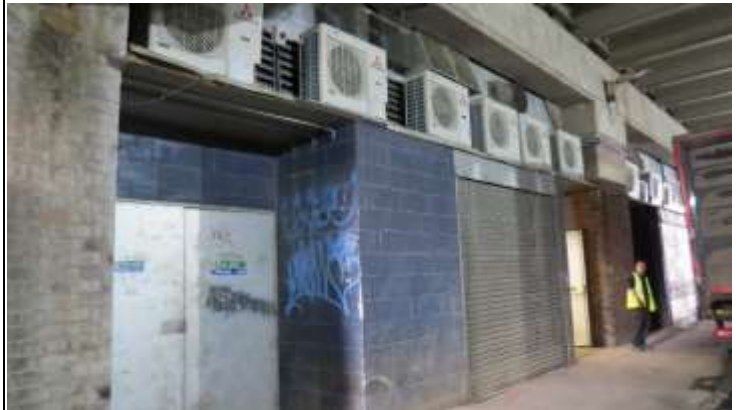
Rear Elevation of Arches 5 and 6
