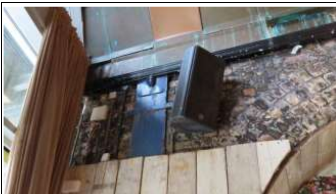
Concealing Boards Between Arches 7 and 8
