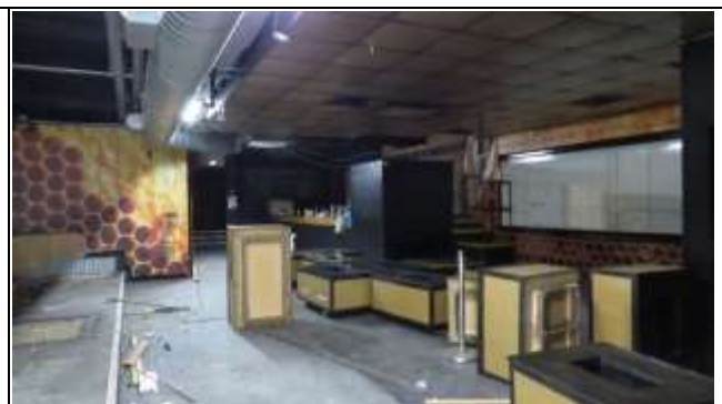
Basement Looking South
