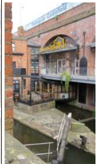
Lock 91, Lock Keepers House and Arch 2
