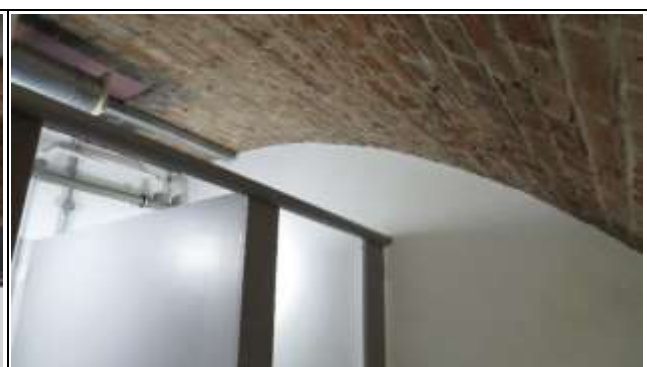
Vaulted Brick Ceiling of Southeast Arch
