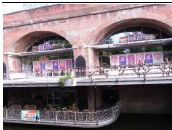
Front Elevation of Arches 9 & 10
