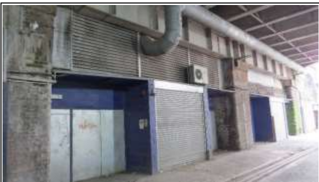
Trafford Street and Rear of West Arches
