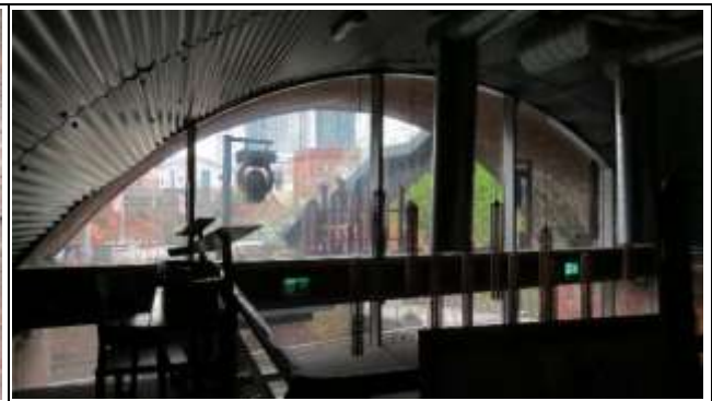
Ceiling of Arch 12 and Mezzanine
