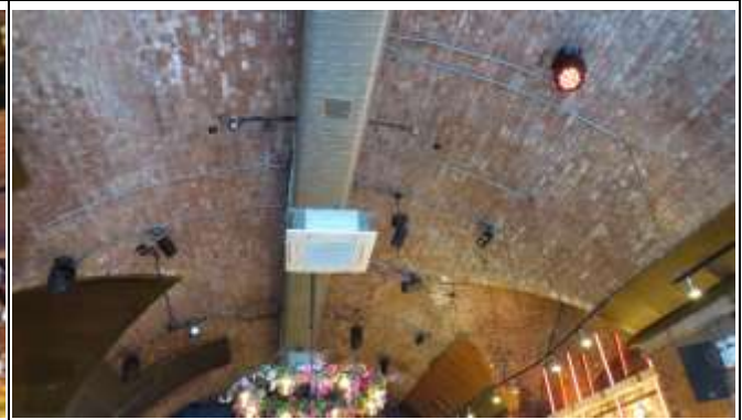
Ceiling of Arch 7
