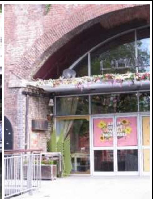
West Interior of Arch 8
