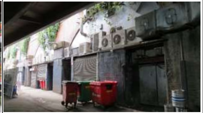
Rear Elevation of Arches 7 and 8
