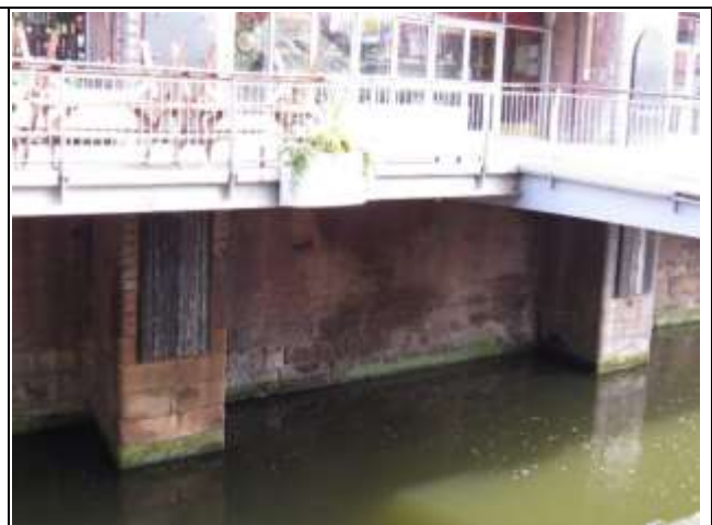
Absence of Basement
