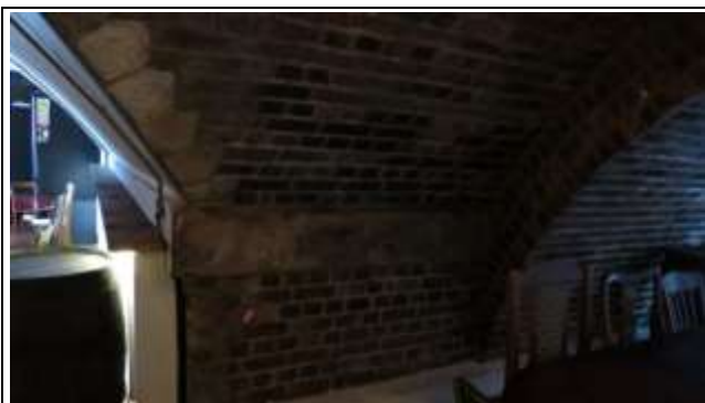
Detail of Arch Brickwork and Impost
