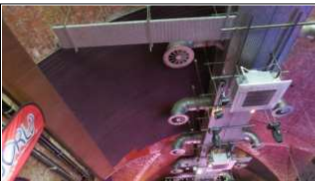
Additional Lining in Arch 6
