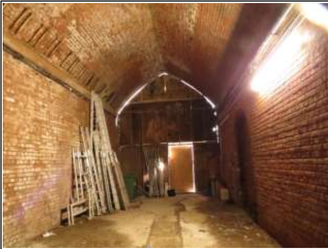
Interior of Arch 1 Rear Storeroom Looking North
