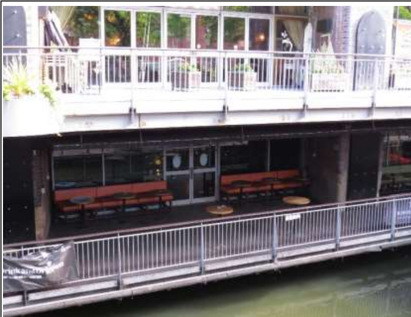
Basement Exterior of Revolution
