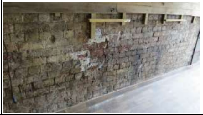
Timber Batons and Wall Lining
