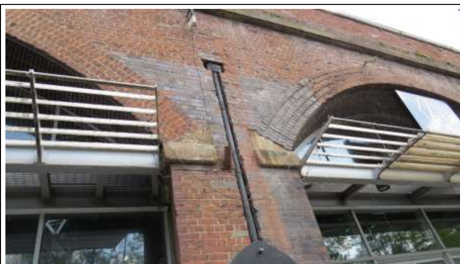
Detail of Arch Brickwork and Rainwater Goods
