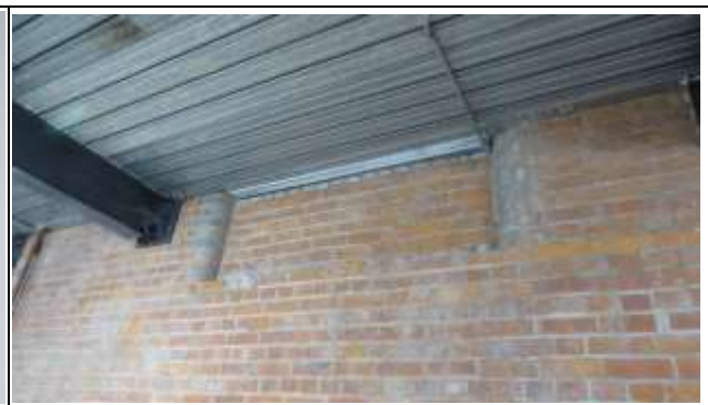
Metal Ceiling and Base of Bricked up Arch
