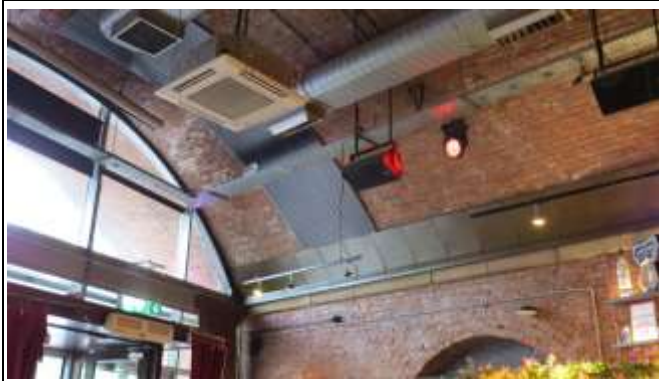
Remedial Works to West Side of Arch 7
