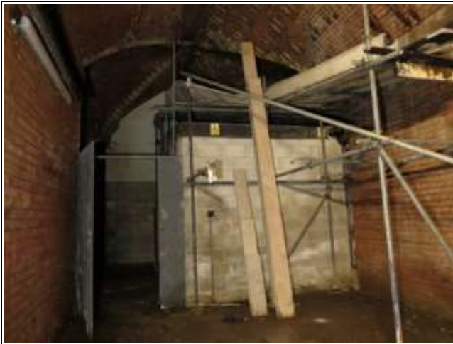
Breezeblock Staircase Structure under Crossvault
