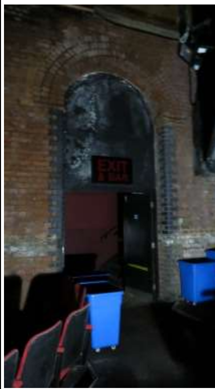
Internal Connecting Arch
