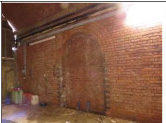
Bricked up Arched Opening to Arch 2
