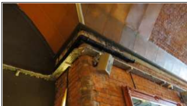
Supplementary Guttering in Ark, Arch 5
