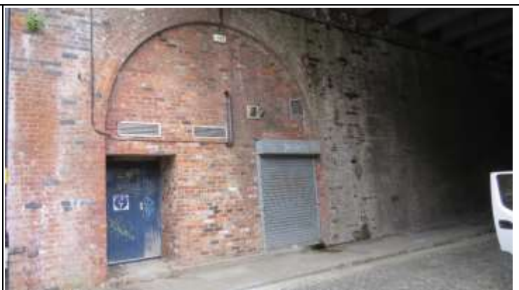
Grey Roller Shutter Entrance to Arch 1 Basement
