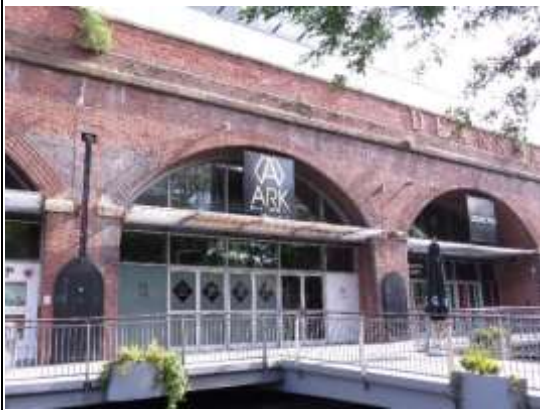
Front Elevation of Arches 5 & 6
