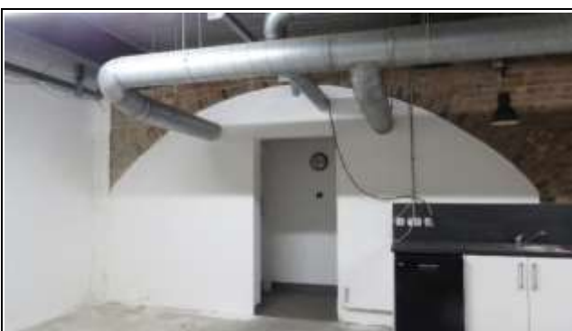
Infilled Arch to Southwest
