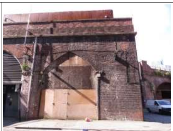
Rear Access to Store off Trafford Street
