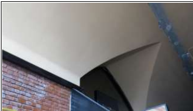
Ceiling Treatment and Gutter
