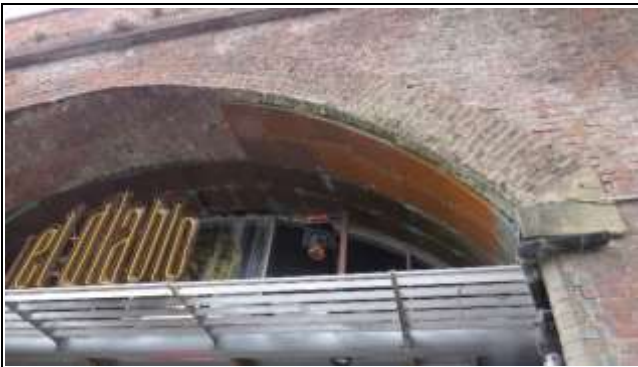
Copper Panels under Arch 11's Entrance
