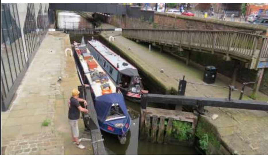
Lock 90 and New Apartment Block
