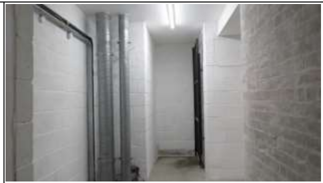
Arch 1 Ancillary Lobby
