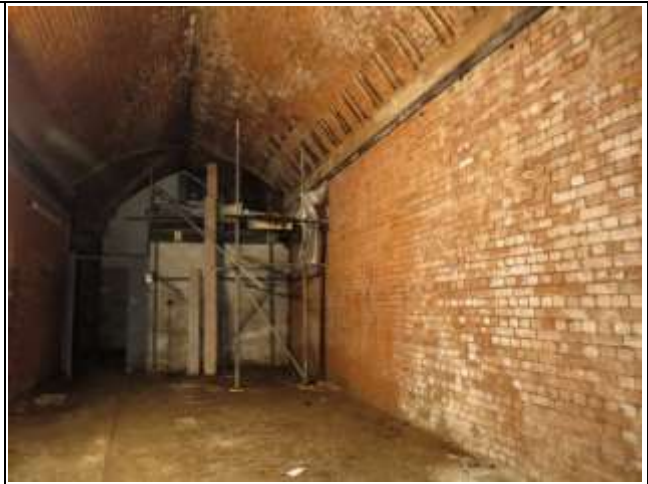
Interior of Arch 1 Rear Storeroom Looking South
