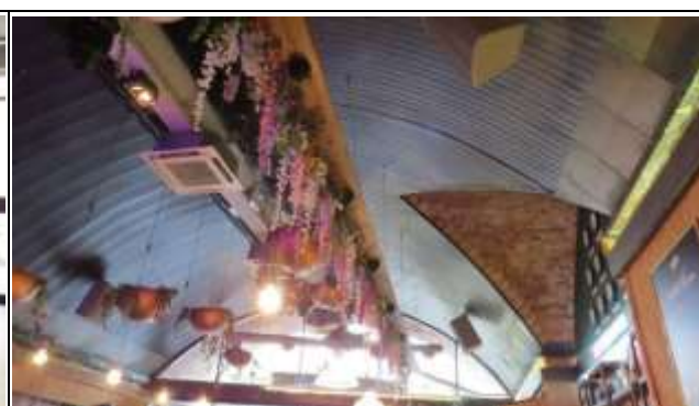
Ceiling to Ground Floor of Arch 9
