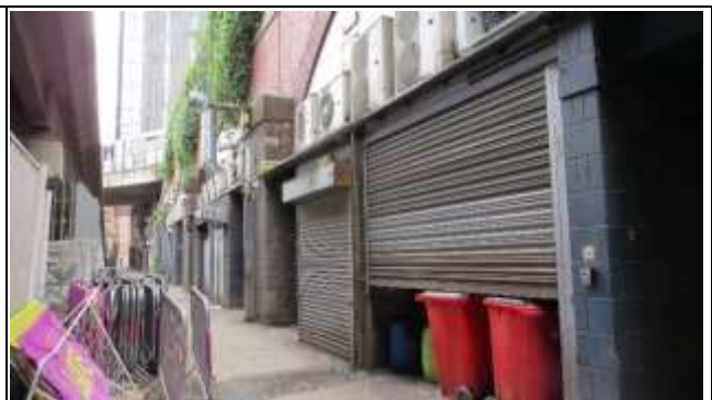
Trafford Street and Rear of East Arches
