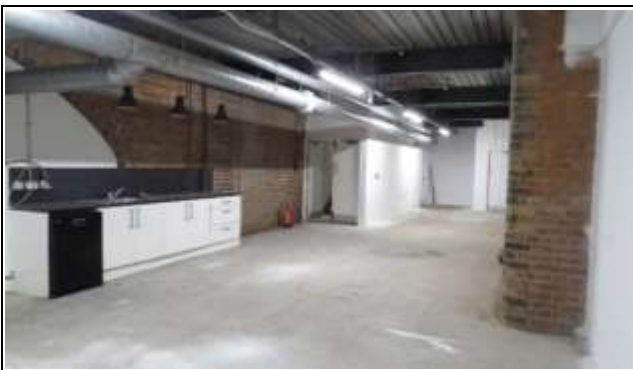
Arch 1 Basement Main Space
