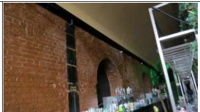
West Wall with Downpipe Attached to Gutter
