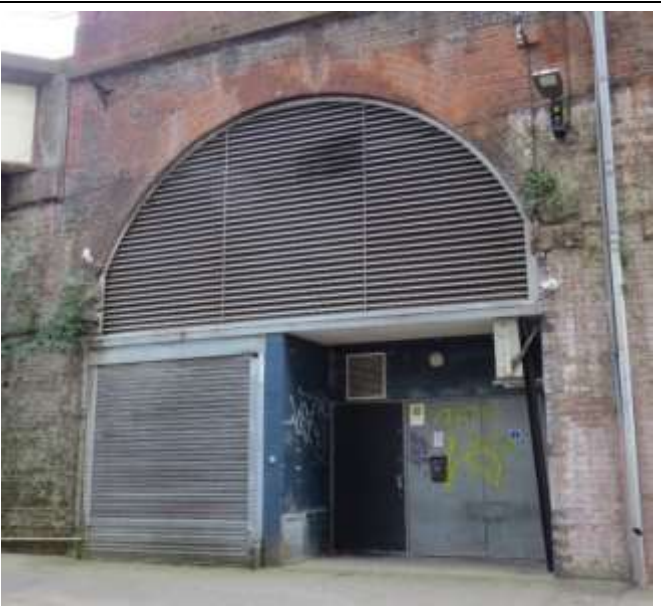
Rear Elevation of Arch 2
