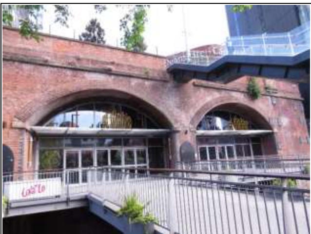
Front Elevation of Arches 11 & 12
