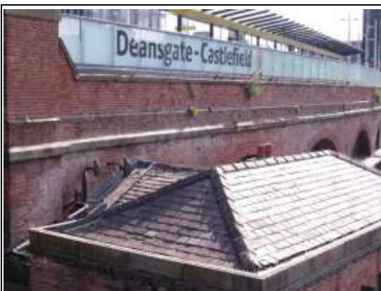
Front of Arch 1 Behind Lock Keeper's House
