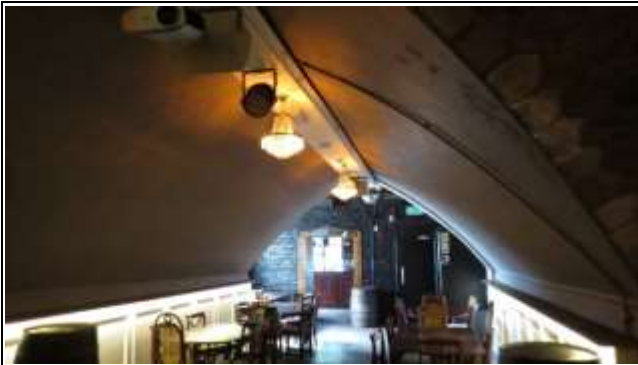
South End of Arch 1 and Lock 91 Beyond
