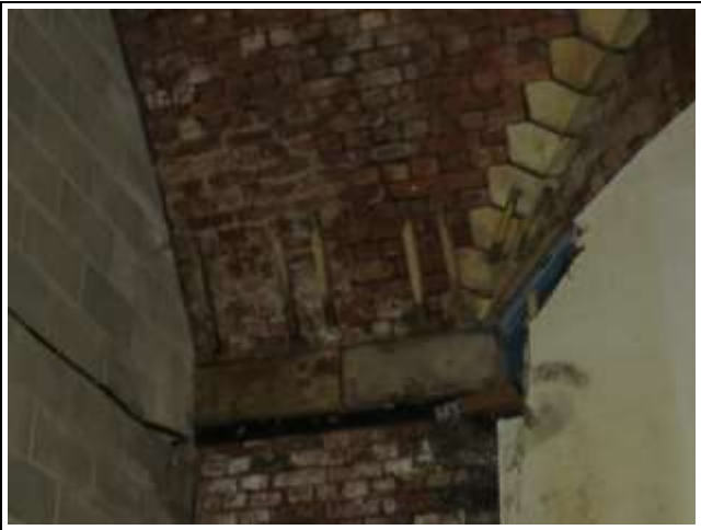
Detail of Blocking up of Crossvault Arches
