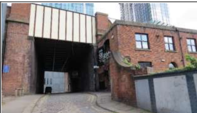
Viaduct with Bridge over Century Street
