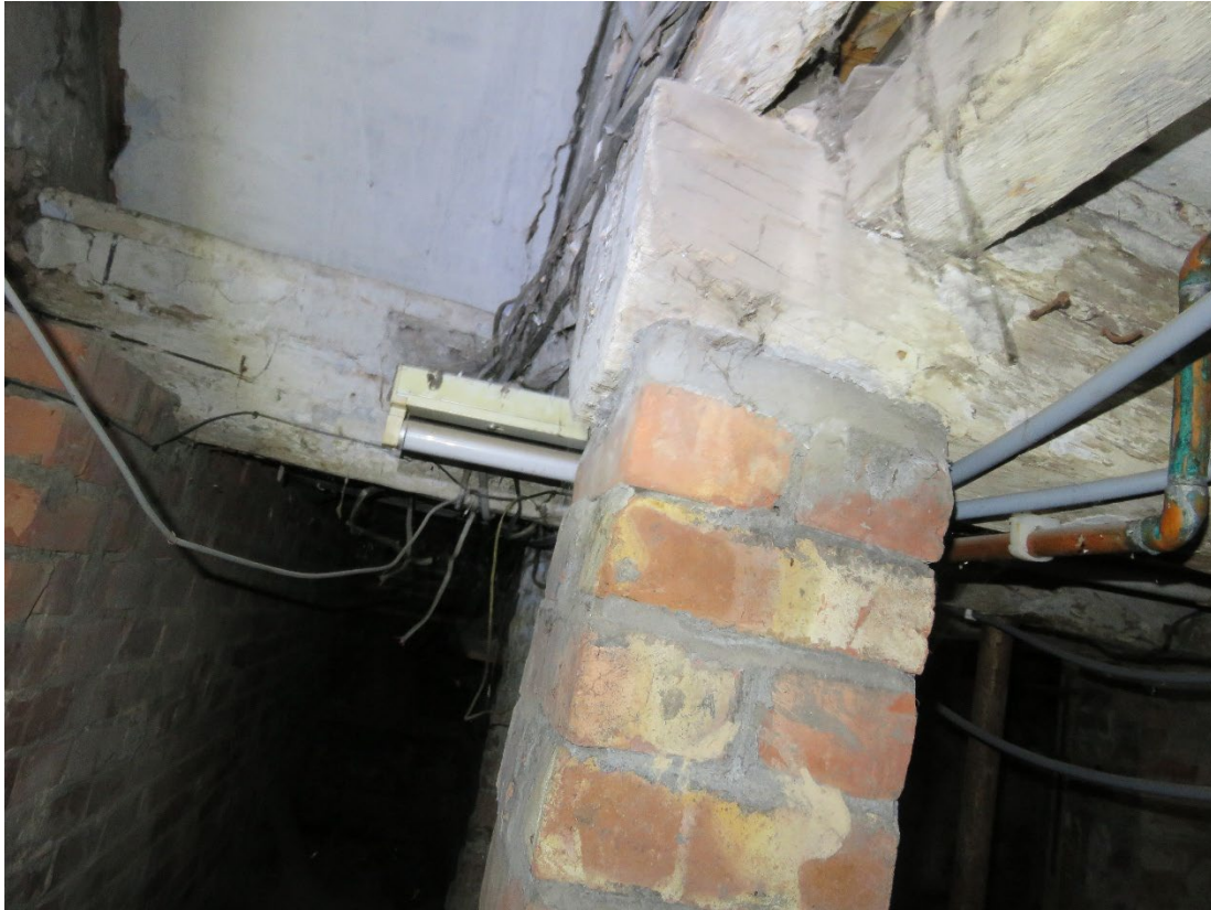
Large oak binder beam in cellar trimmed back in the past, supported by a brick pillar.
