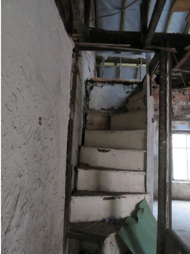
Existing attic staircase.
