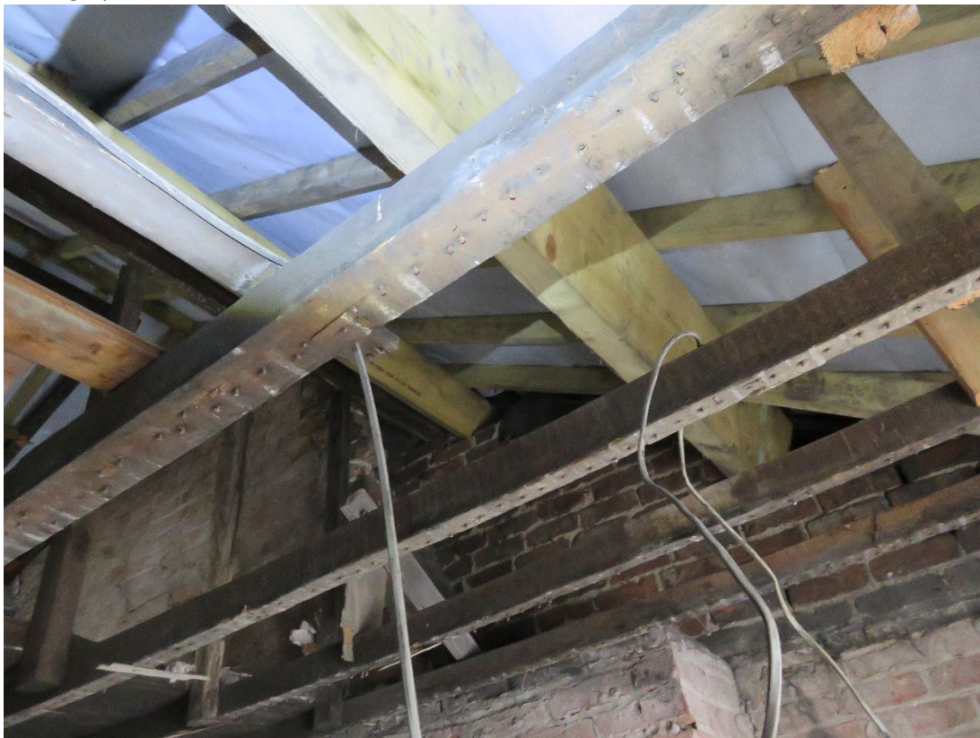
New timber purlin.
