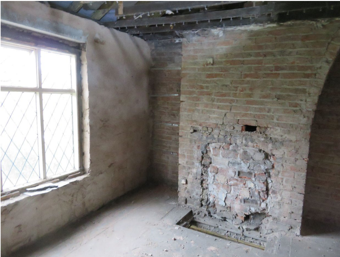
Front binder beam to chimney breast to be replaced. Party wall lateral restraint strap previously installed.
