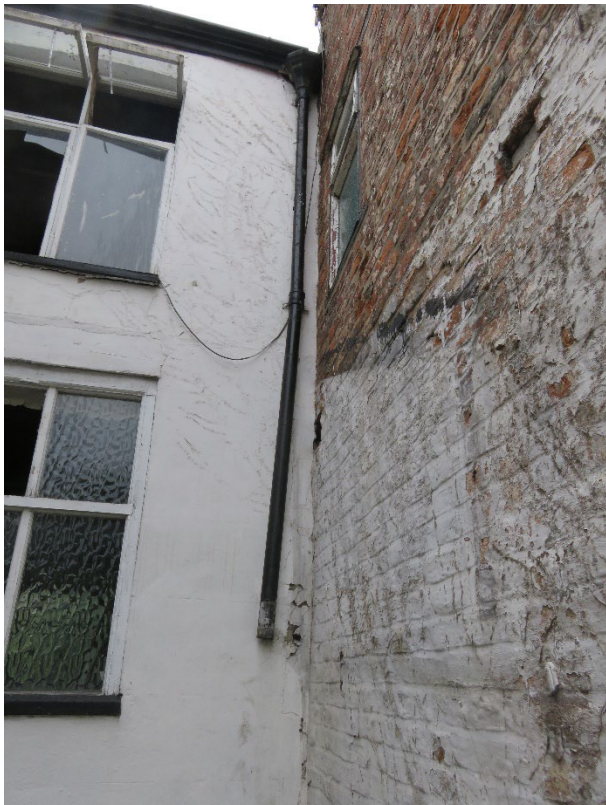
Extend rainwater pipe in cast iron.
