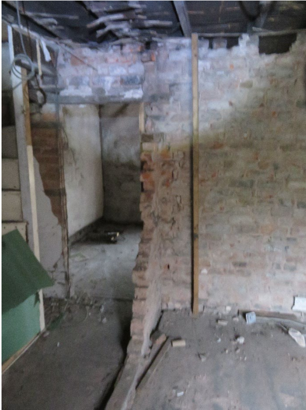
Wall to be rebuilt in reclaimed brickwork.
