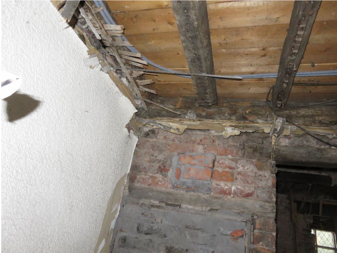
Open up old opening staircase from cellar.
