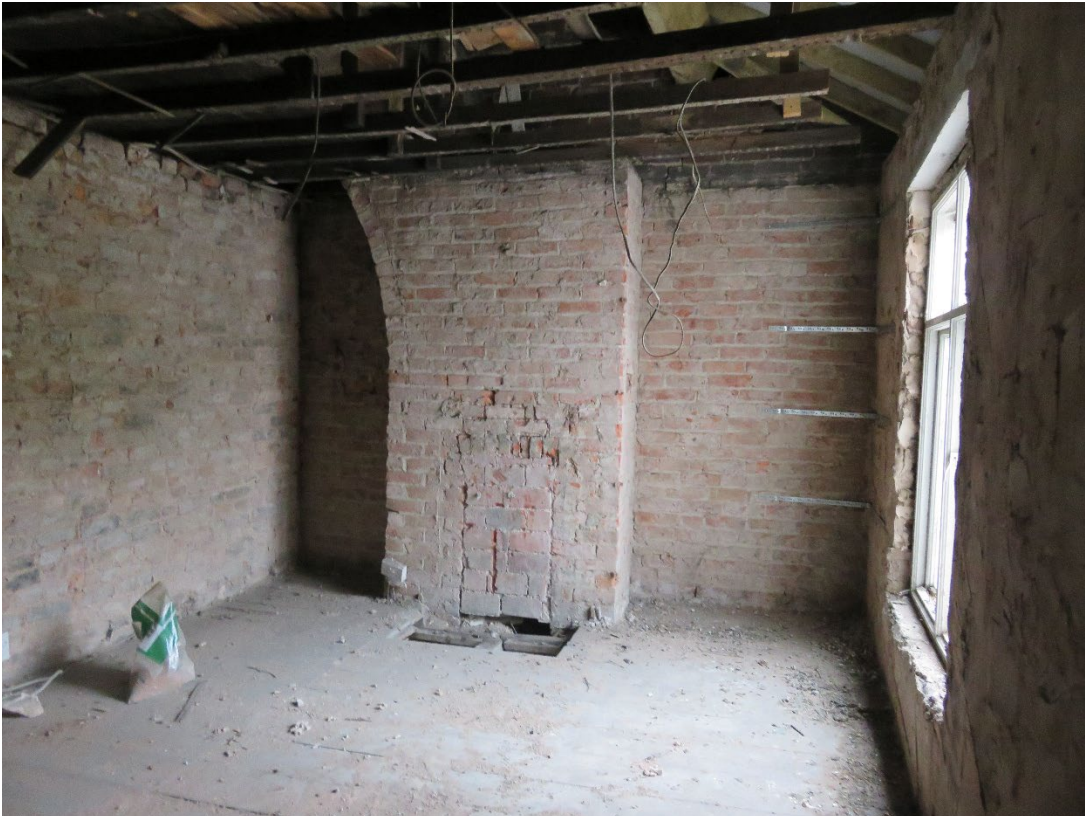
Built up chimney breast.
