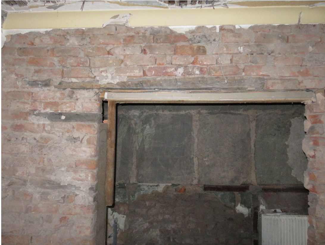
Reposition door as under original lintel.
