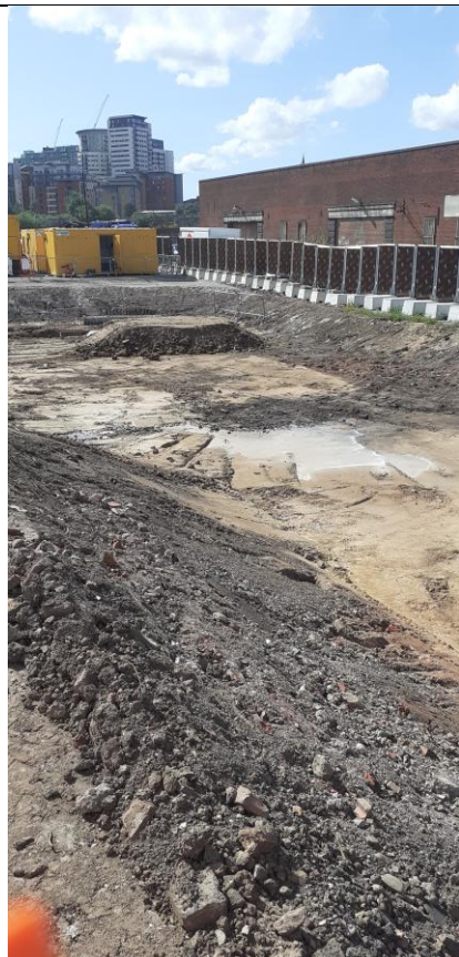
Excavated area within NT04 – minor ponding of water
