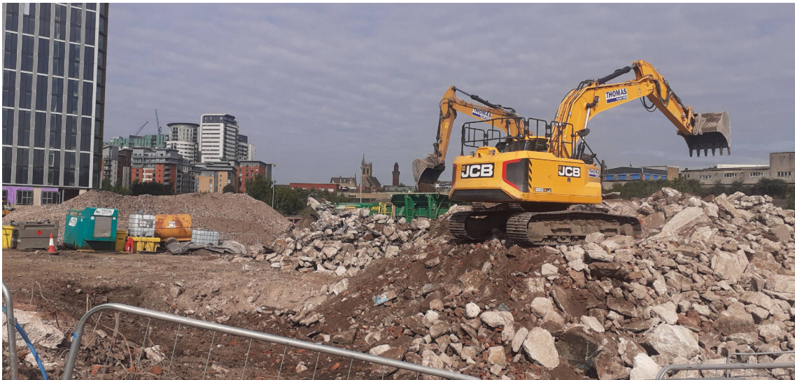
NT03 Concrete crushing / grading on going
