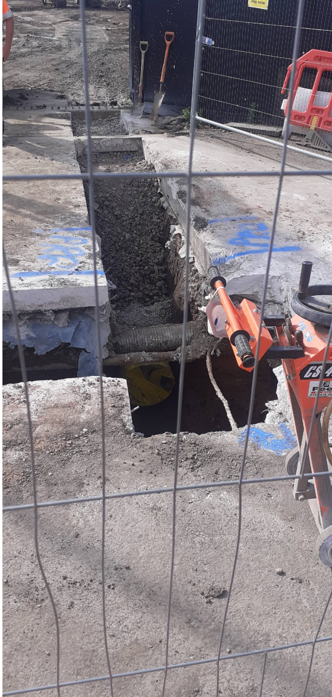
Diverted gas main at Road, main trench infilled
