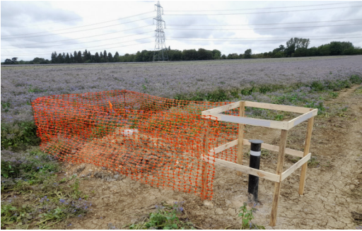
Example 1 : Fenced in well enclosure
