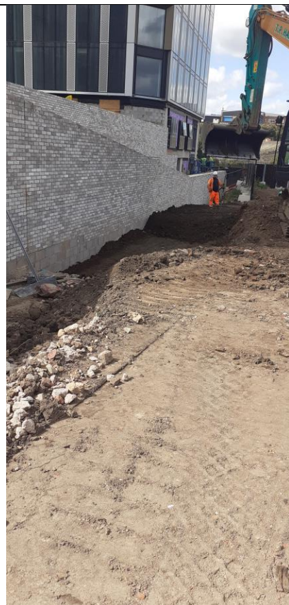
Backfilling to boundary wall – NT02
