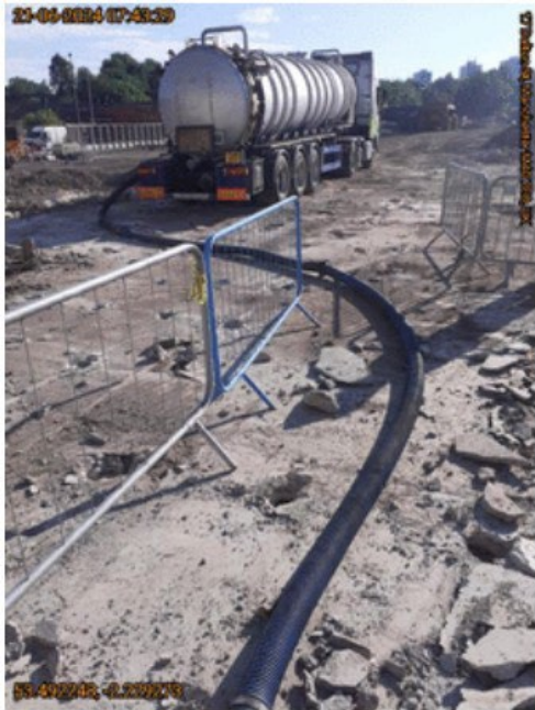
NT02 Tankering off of contents
