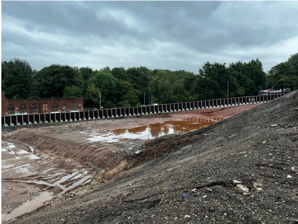
Network Rail Mound Piling Platform
