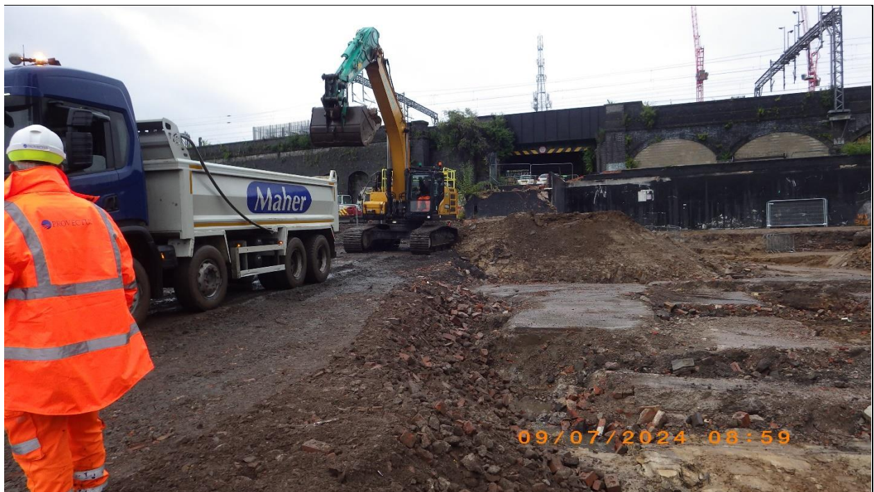
Second round of excavation works: soils being loaded from TCE
