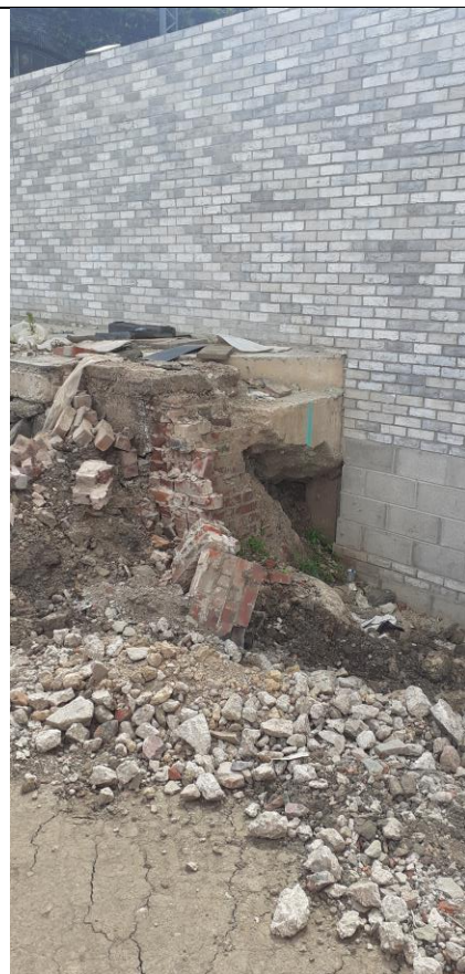
Backfilling to boundary wall – NT02 Foundations to be covered with backfill
