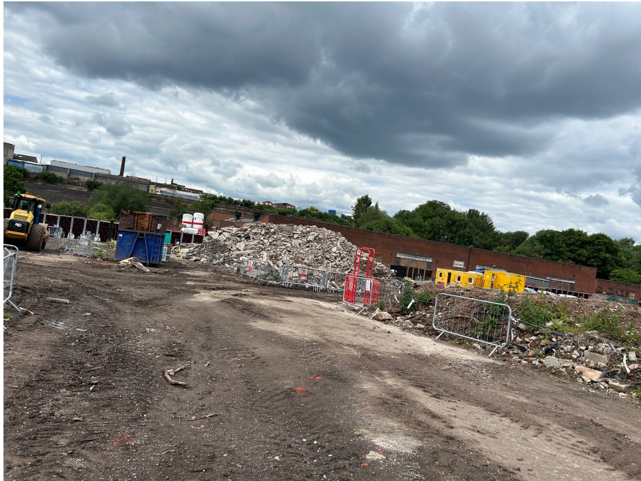
NT02 Slab broken out and surface compacted
