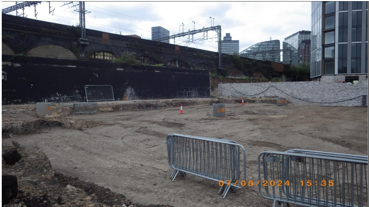
Facing south, TCE area post-upfill. Concrete rings now placed around BHs
