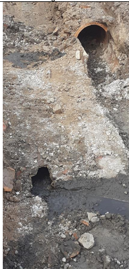
375mm dia SW pipe with approx. 225mm dia additional pipe found adjacent
