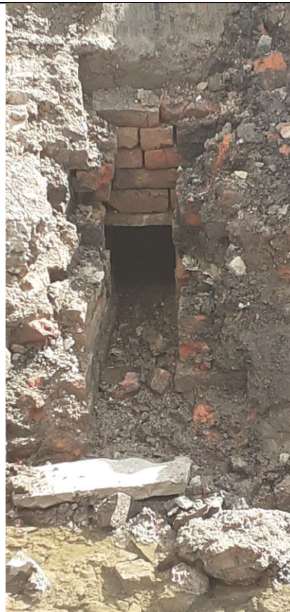
Brick culvert – CCTV received from BAM 27.08.2024
