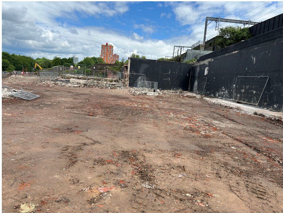
NT02 Slab broken out and surface compacted
