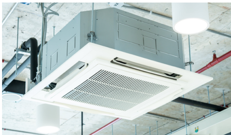
Example of an exposed ceiling mounted AC unit.
