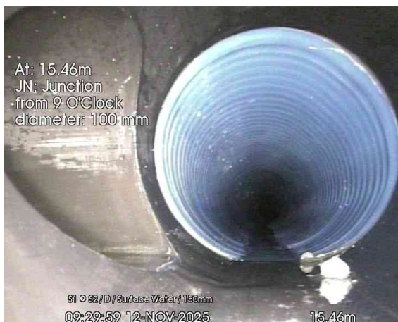
3, 00:01:02, 15.46 m Junction at 9 o'clock, 100mm dia
