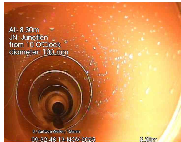
6, 00:00:45, 8.30 m Junction at 10 o'clock, 100mm dia
