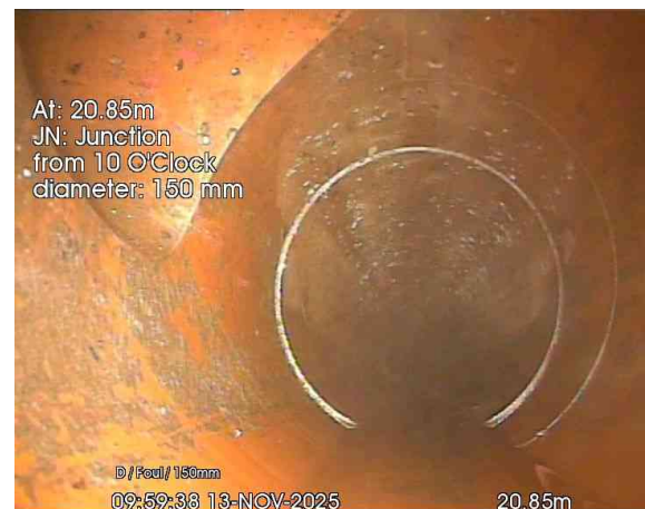
4, 00:01:11, 20.85 m Junction at 10 o'clock, 150mm dia
