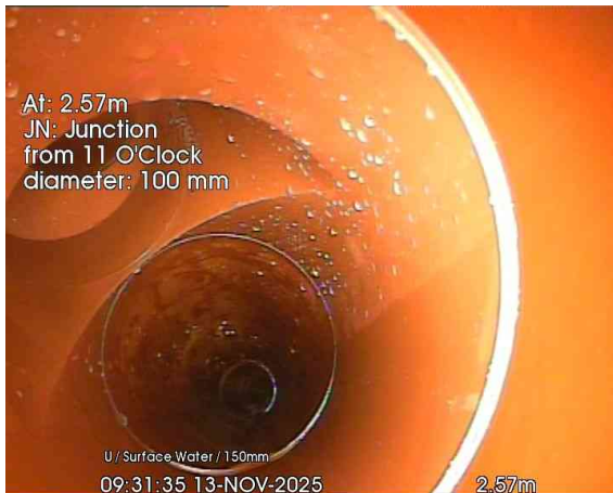
1, 00:00:21, 2.57 m Junction at 11 o'clock, 100mm dia
