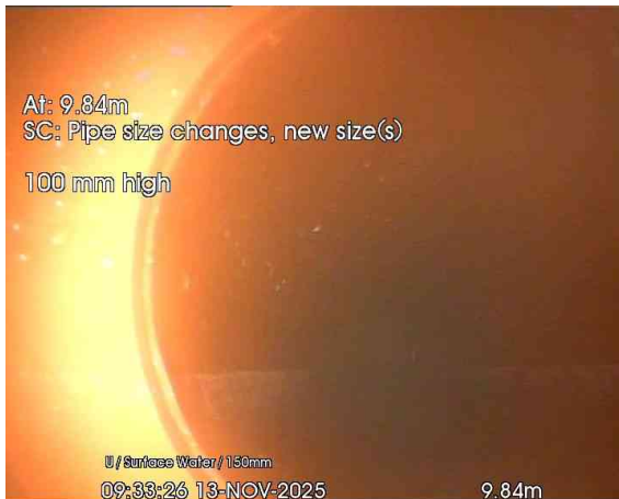
9, 00:00:57, 9.84 m Pipe size changes, new size(s), 100mm high
