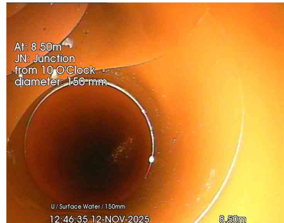
2, 00:00:24, 8.50 m Junction at 10 o'clock, 150mm dia
