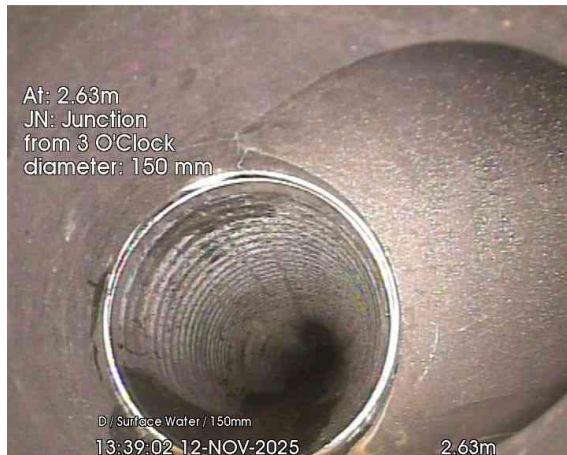
1, 00:00:13, 2.63 m Junction at 3 o'clock, 150mm dia
