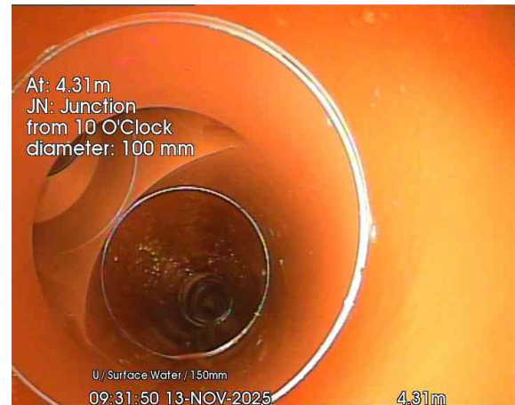
2, 00:00:28, 4.31 m Junction at 10 o'clock, 100mm dia
