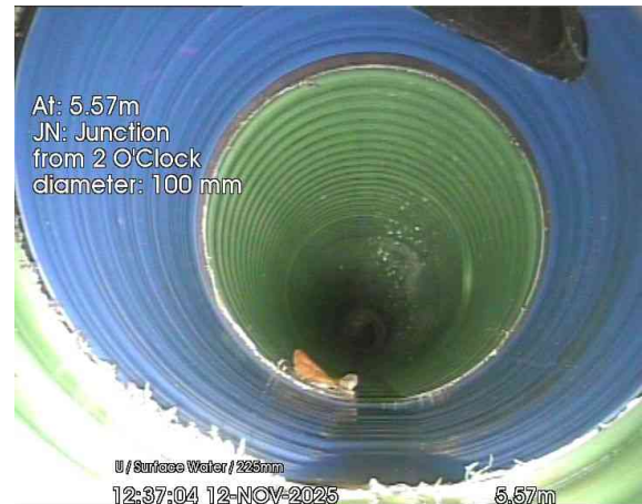
2, 00:00:41, 5.57 m Junction at 2 o'clock, 100mm dia
