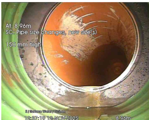
3, 00:00:49, 8.96 m Pipe size changes, new size(s), 150mm high
