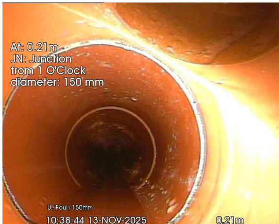
1, 00:00:07, 0.21 m Junction at 1 o'clock, 150mm dia
