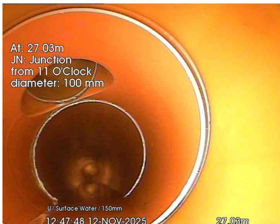
5, 00:01:15, 27.03 m Junction at 11 o'clock, 100mm dia
