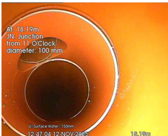
3, 00:00:46, 18.19 m Junction at 11 o'clock, 100mm dia
