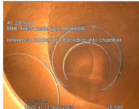
6, 00:01:41, 28.90 m Finish node, manhole, reference: C1, Backdrop into chamber
