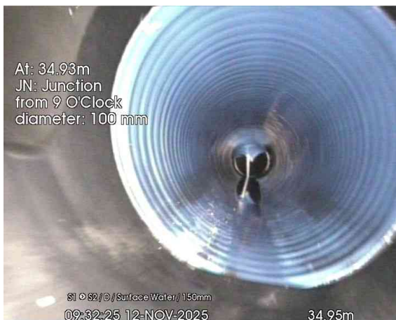
7, 00:02:22, 35.06 m Junction at 9 o'clock, 100mm dia
