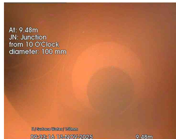
8, 00:00:55, 9.48 m Junction at 10 o'clock, 100mm dia
