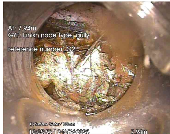
2, 00:00:47, 7.94 m Finish node, gully, reference: G2
