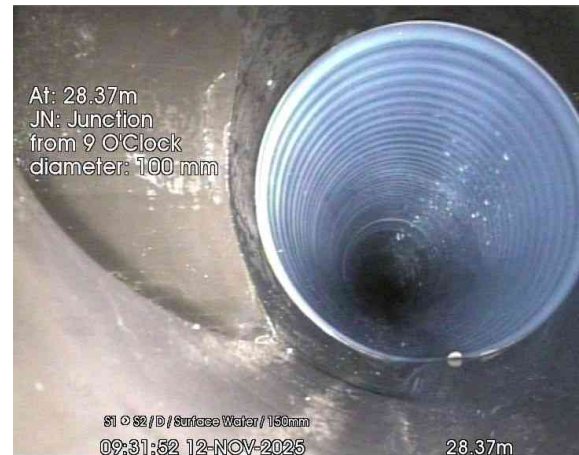
6, 00:02:02, 28.37 m Junction at 9 o'clock, 100mm dia
