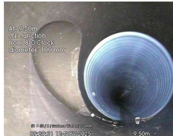
2, 00:00:43, 9.50 m Junction at 8 o'clock, 100mm dia
