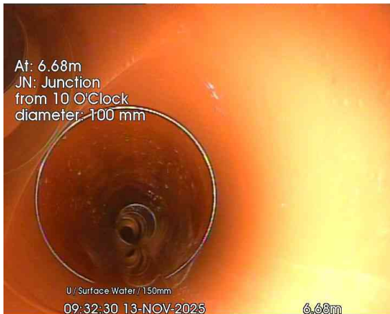
5, 00:00:39, 6.68 m Junction at 10 o'clock, 100mm dia
