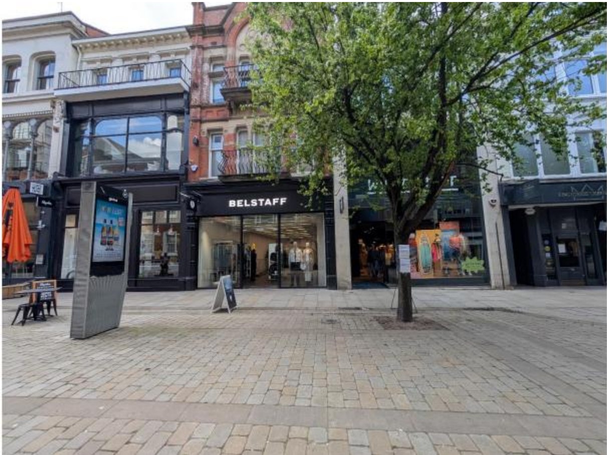
(Figure 15: Application site along King Street, within Primary Shopping Area/Retail Core)
