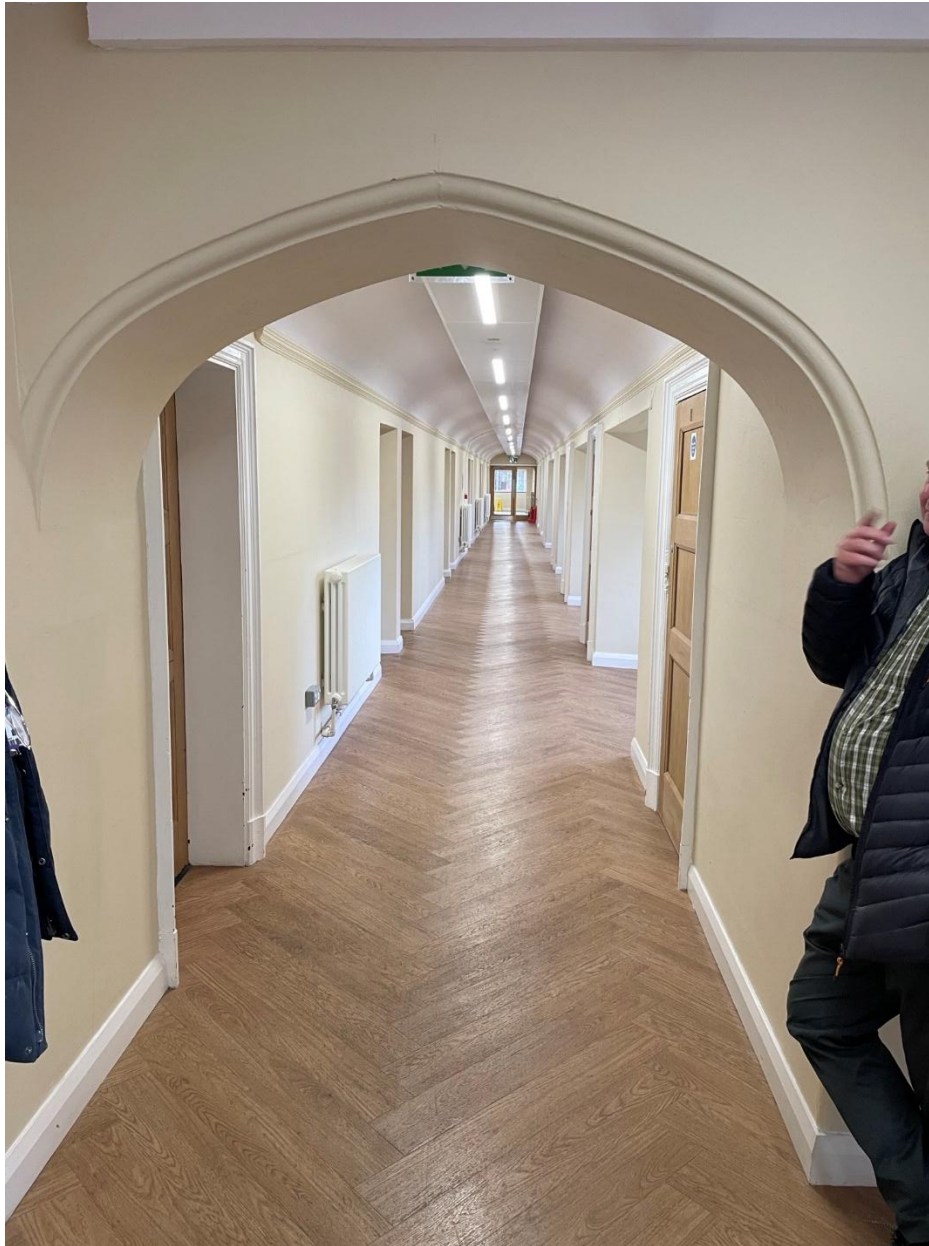
Photo 2. Location for proposed new cross corridor door outside the kitchen on the first floor. Door to fit in existing archway and to match door in Photo 1.
