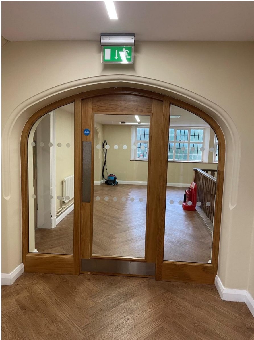
Photo 1. Existing timber framed glass door with glass panel on either side. Door is located to stairway on the first floor of Houldsworth Hall.
