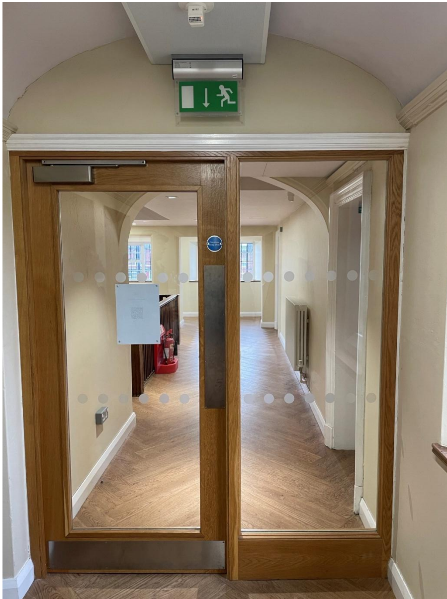
Photo 3. Existing timber framed glass door with glass panel on the right-hand side. Door is located to stairway on the first floor of Houldsworth Hall.
