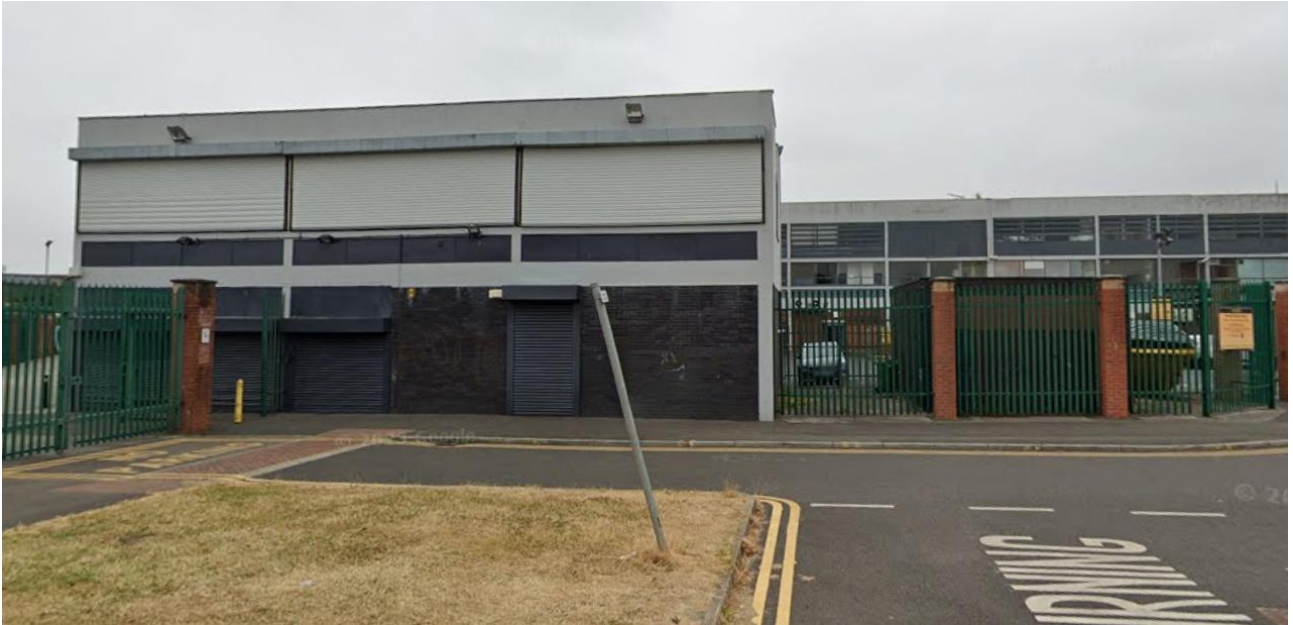
Plate B.1 Northwest elevation of building from the adjacent road
