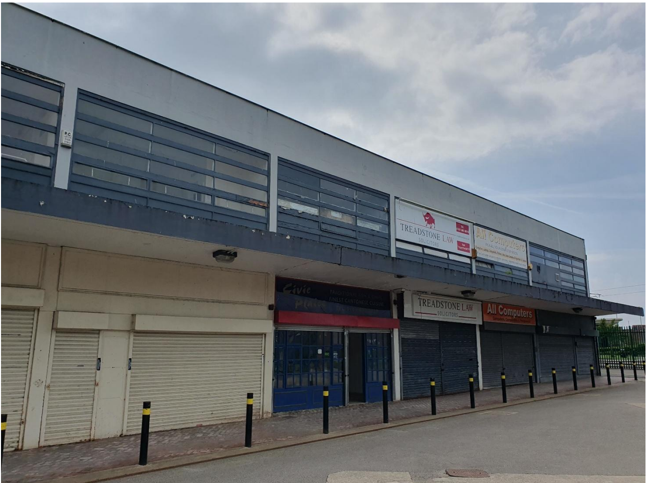
Plate B.2 Northern elevation, rows of previously used commercial units are present
