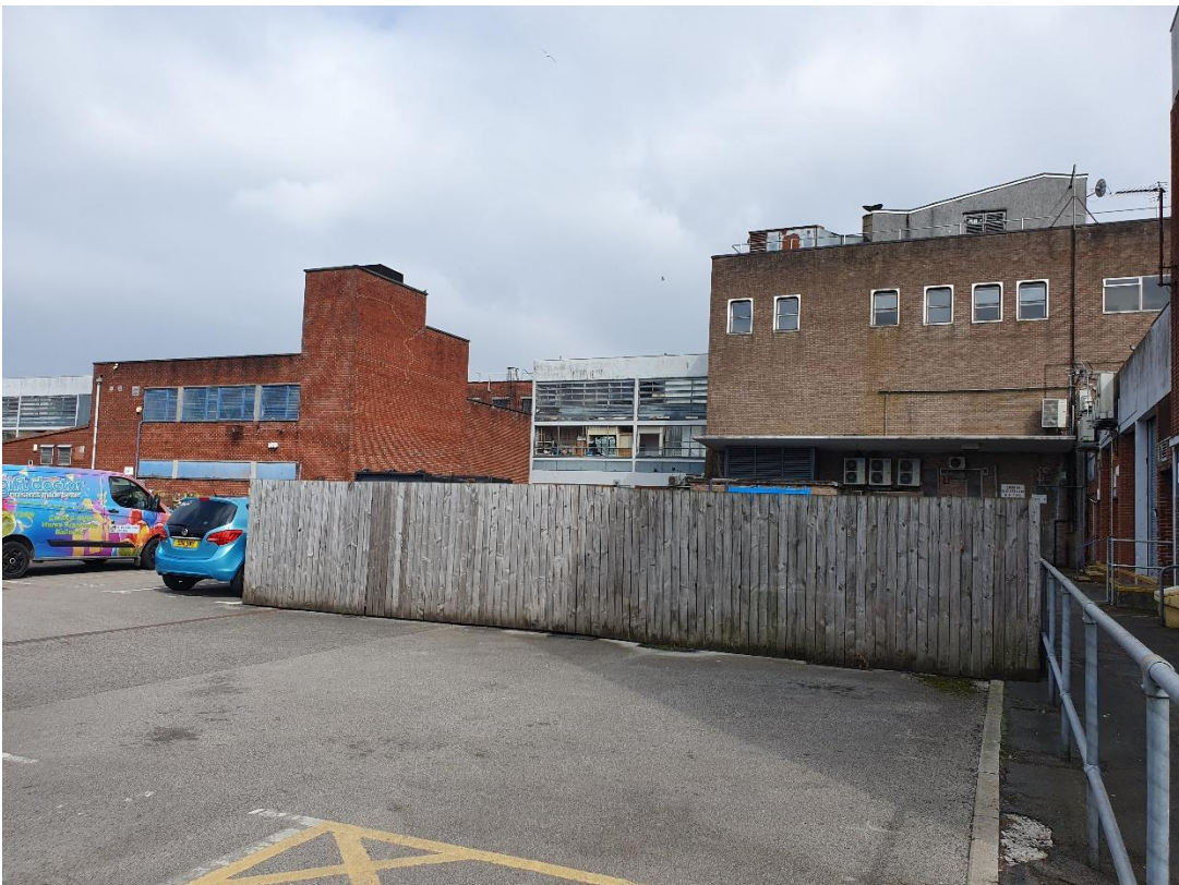
Plate B.4 Southern area of the site, the adjacent market 'The Birtles' can be seen over the fence
