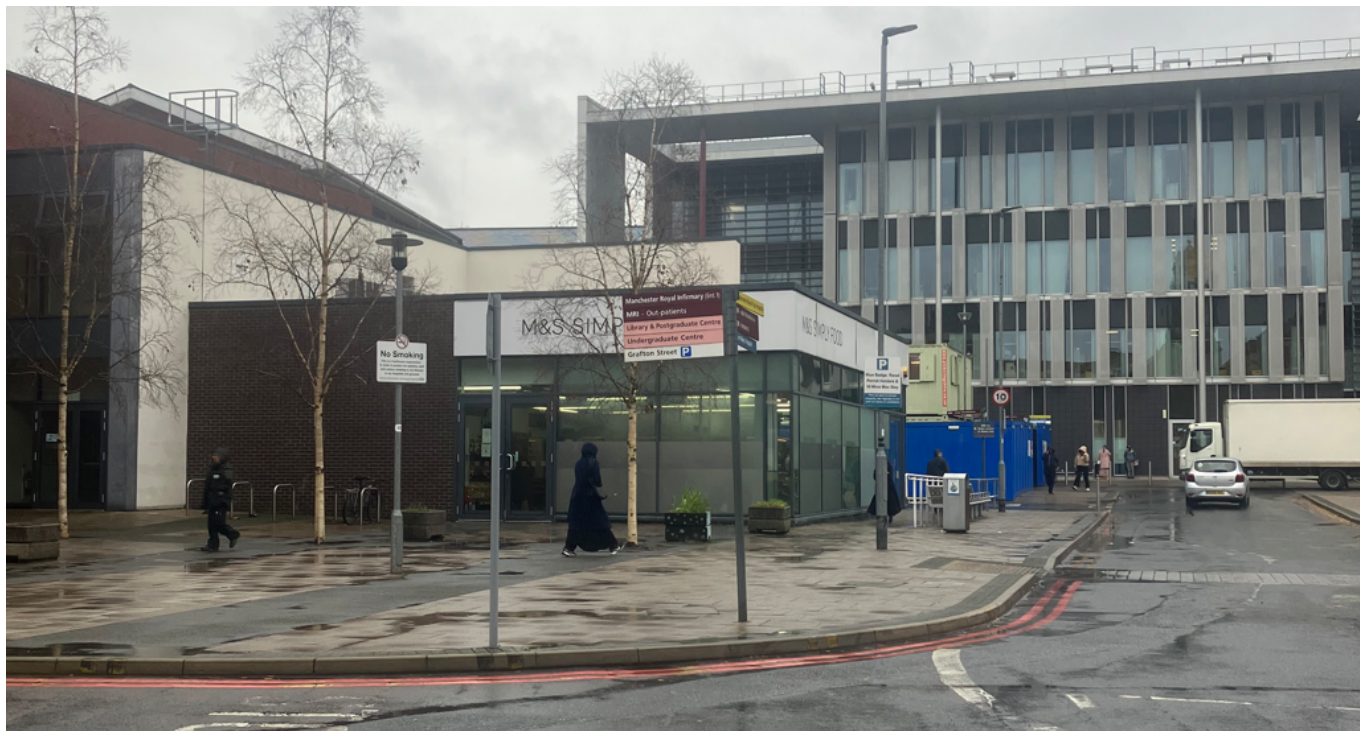
The application site (foreground) and MRI building (background).
