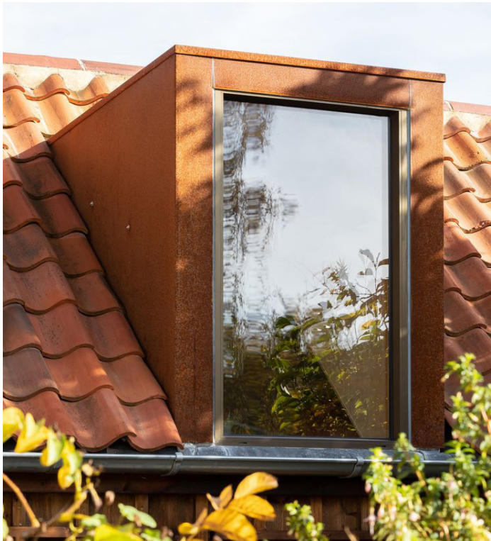
Clay Tile Mansard Roof with Flat Dormer
