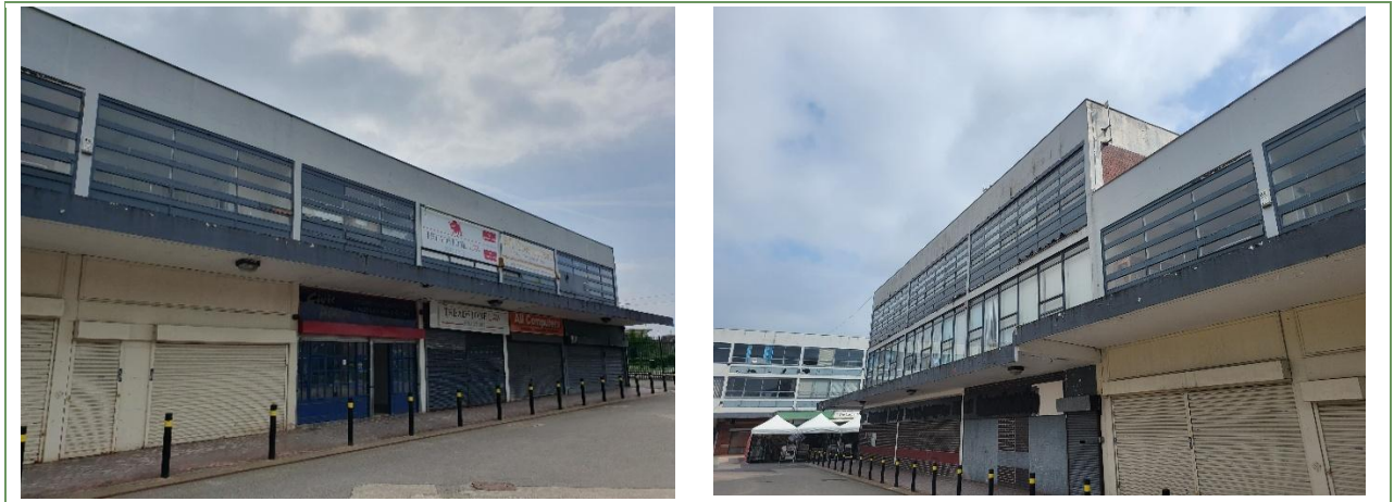
Plate C.1 Northern aspect of the building (right and left)
