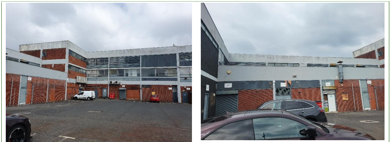
Plate C.2 Western aspect (left) and southern aspect (right) of the building from the internal car parking
