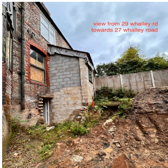
View to 27 Whalley Rd at basement level
