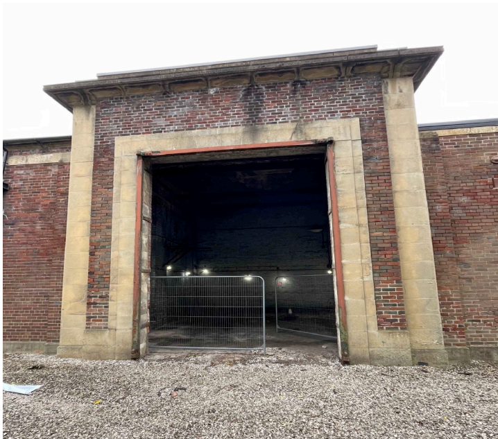
Photo 3: existing front elevation of the sub station
