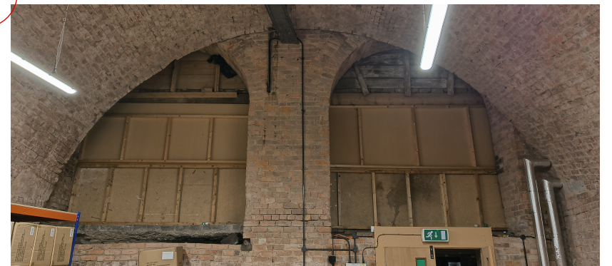
Photo 2 SIM.SB.-1.16 PINs A1SB-116A and A1SB-116B
