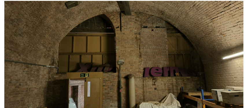
Photo 1 SIM.SB.-1.15 PINs A1SB-115A and A1SB-115B
