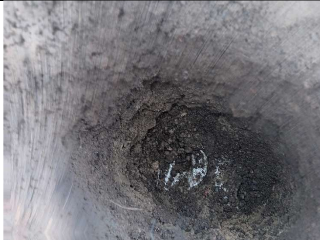
View of soil in capping layer excavation in soft landscaping. Demarcation membrane at base.
