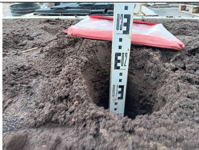
Depth measurement HD114 ( circa 290mm soil cover over membrane).
