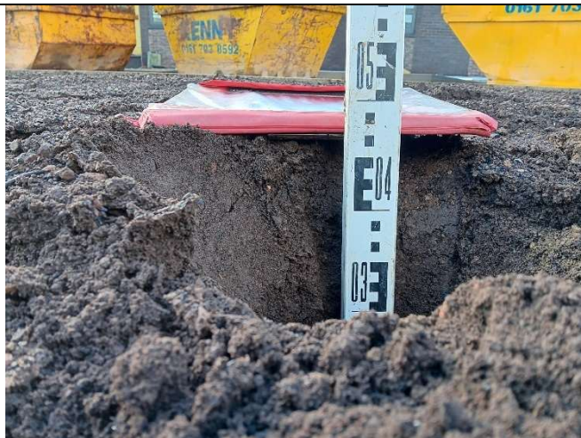
Depth measurement HD102 ( circa 470mm soil cover over membrane ).
