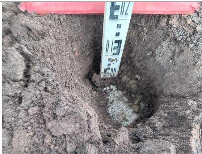
View of soil in capping layer excavation in soft landscaping. Demarcation membrane at base.
