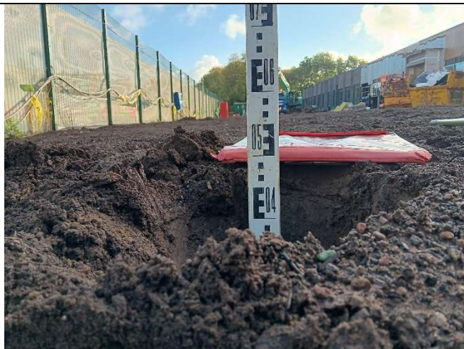
Depth measurement HD101 ( circa 490mm soil cover over membrane).
