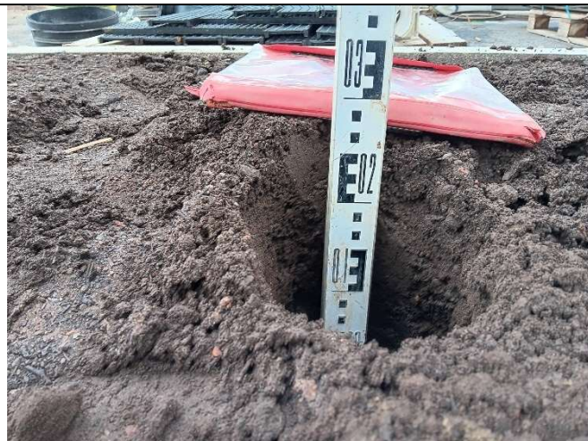
Depth measurement HD115 ( circa 280mm soil cover over membrane).
