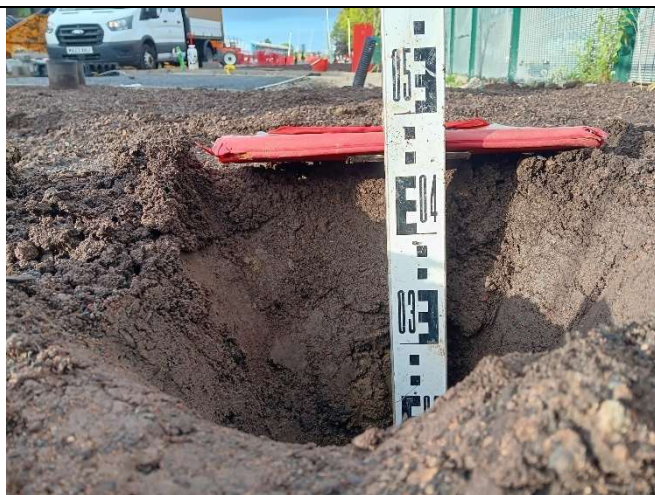
Depth measurement HD103 ( circa 470mm soil cover over membrane).
