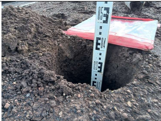
Depth measurement HD119 ( circa 450mm soil cover over membrane).
