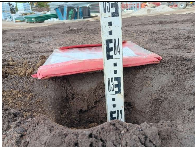
Depth measurement HD113 ( circa 380mm soil cover over membrane).
