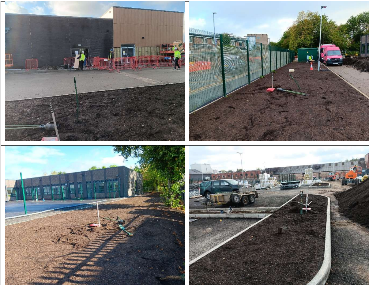
Photographs 1-4: Selected photographs of completed site.
