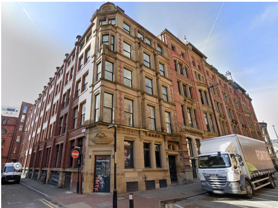
Figure 1. Application Site (Google Maps, 2022)
