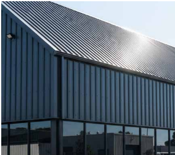
Corrugated metal roof and cladding
