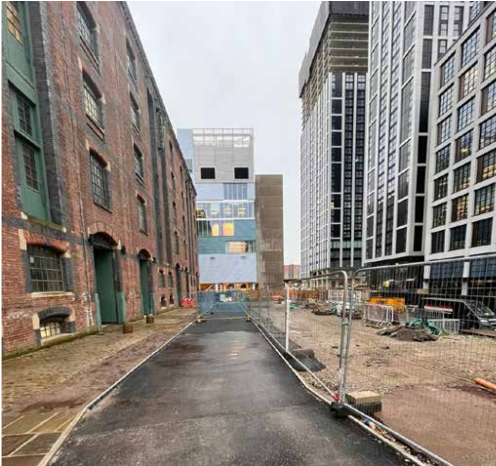
View looking west, towards The Factory
