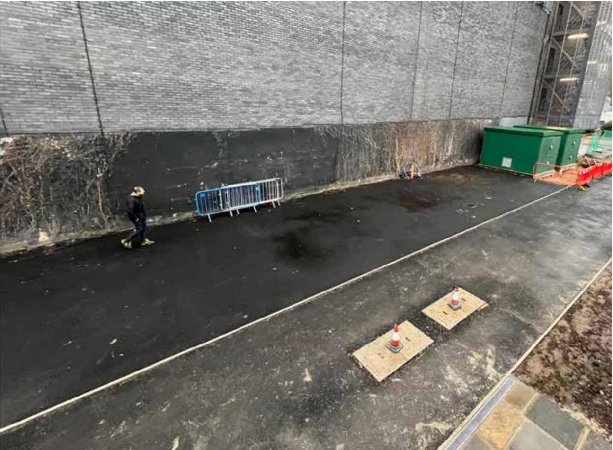
View looking east, showing the existing substations
