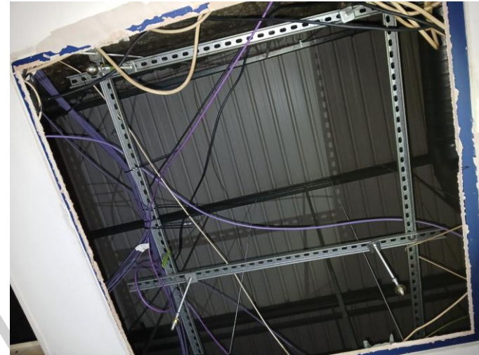
B1 – Internal roof structure
