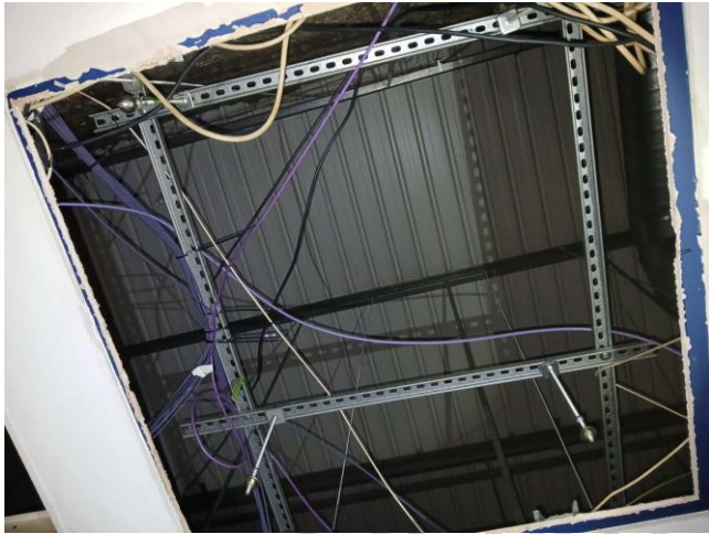
Photo 33: View of internal roof structure
