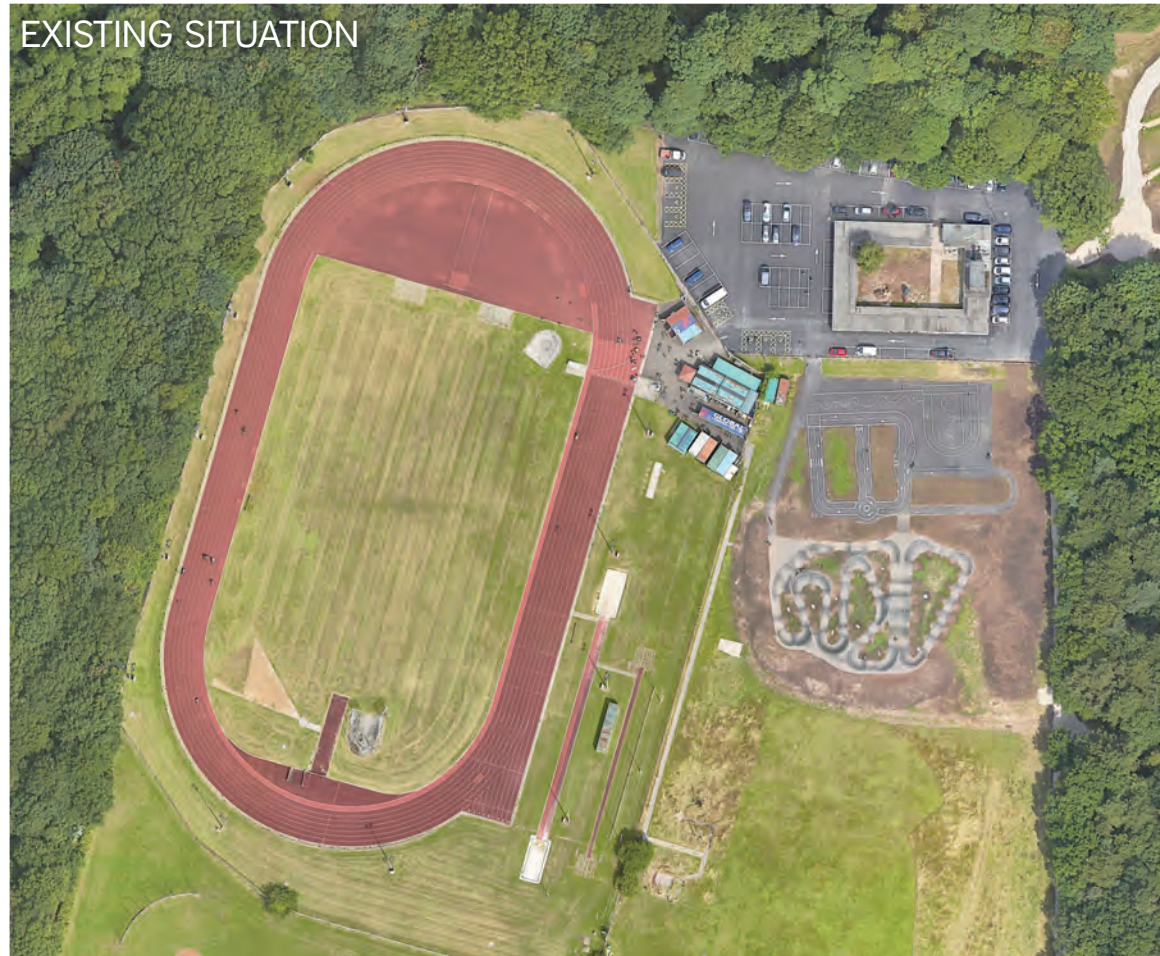
Fig 2 - Existing situation at the Wythenshawe Park Sport Hub Site.
