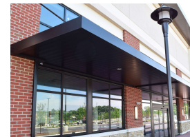
6. Feature Cantilever Canopy (Finish to match glazing)
