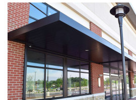
6. Feature Cantilever Canopy (Finish to match glazing)
