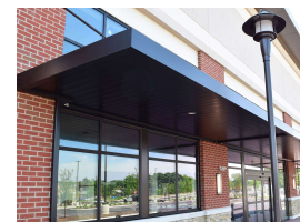
6. Feature Cantilever Canopy (Finish to match glazing)
