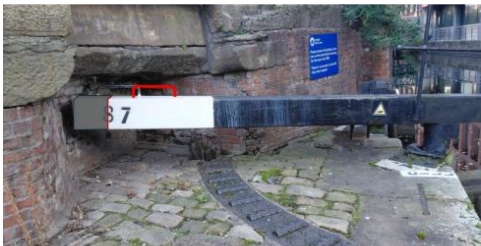
Figure 4 – Shortening of balance beam
