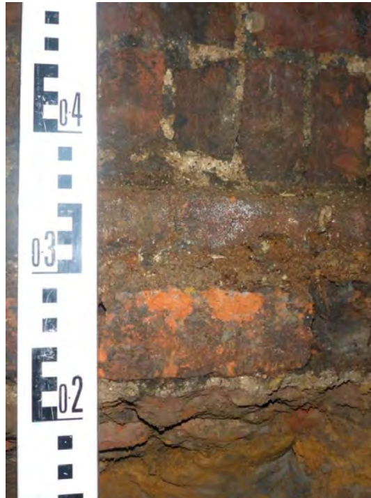
Trial Pit JTP06 - Photo 23
