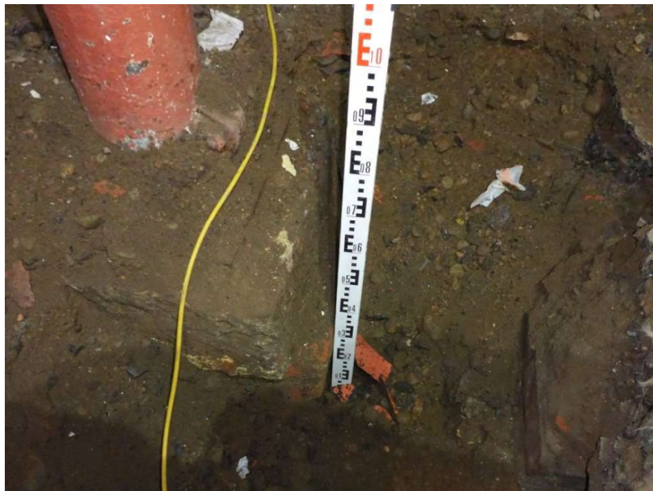
Trial Pit JTP02 - Photo 2
