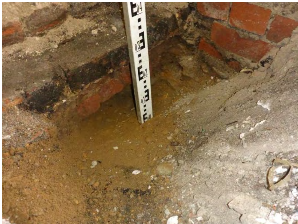
Trial Pit JTP05 - Photo 2
