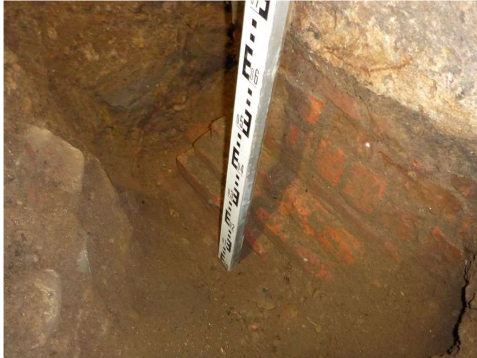
Trial Pit JTP02 - Photo 2
