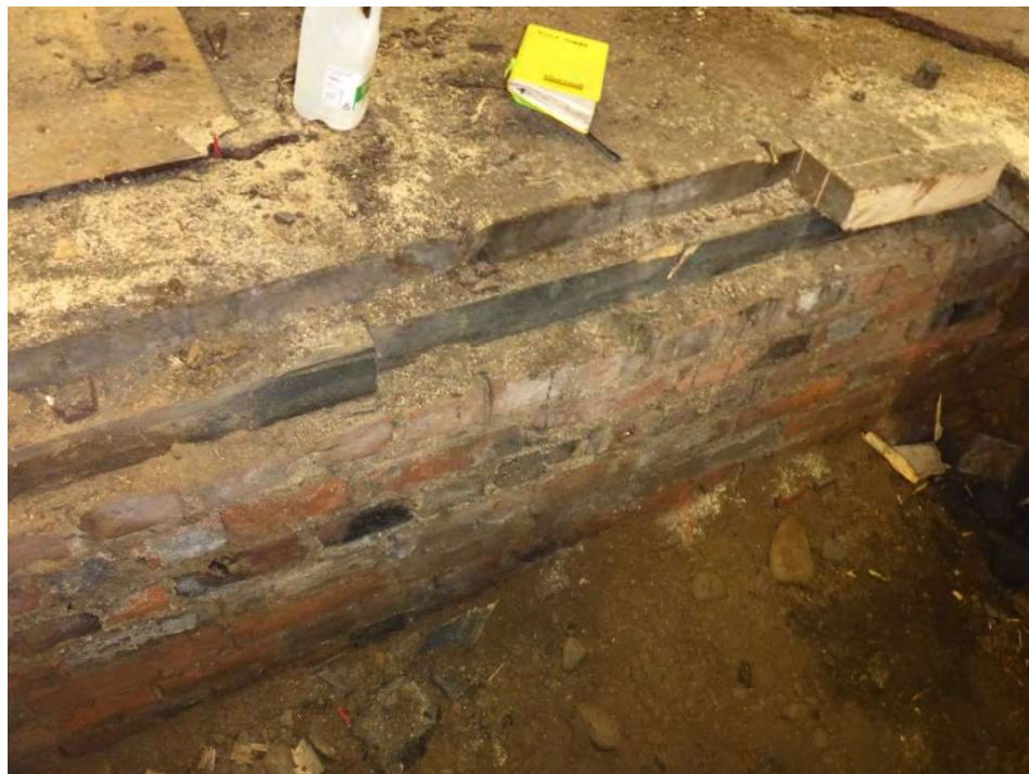
Trial Pit JTP02 - Photo 3
