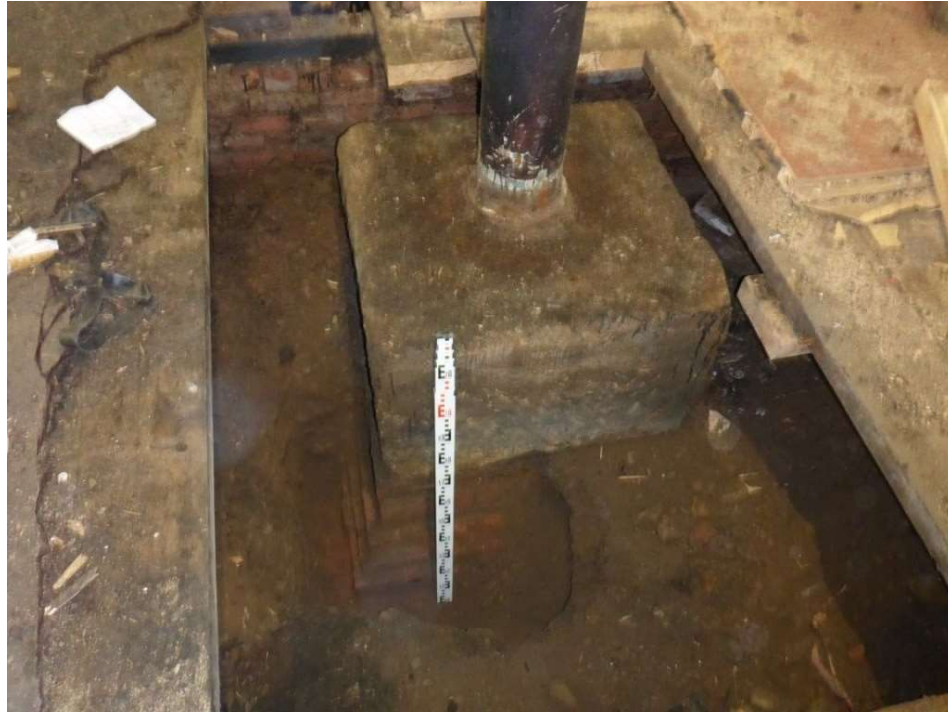
Trial Pit JTP02 - Photo 1
