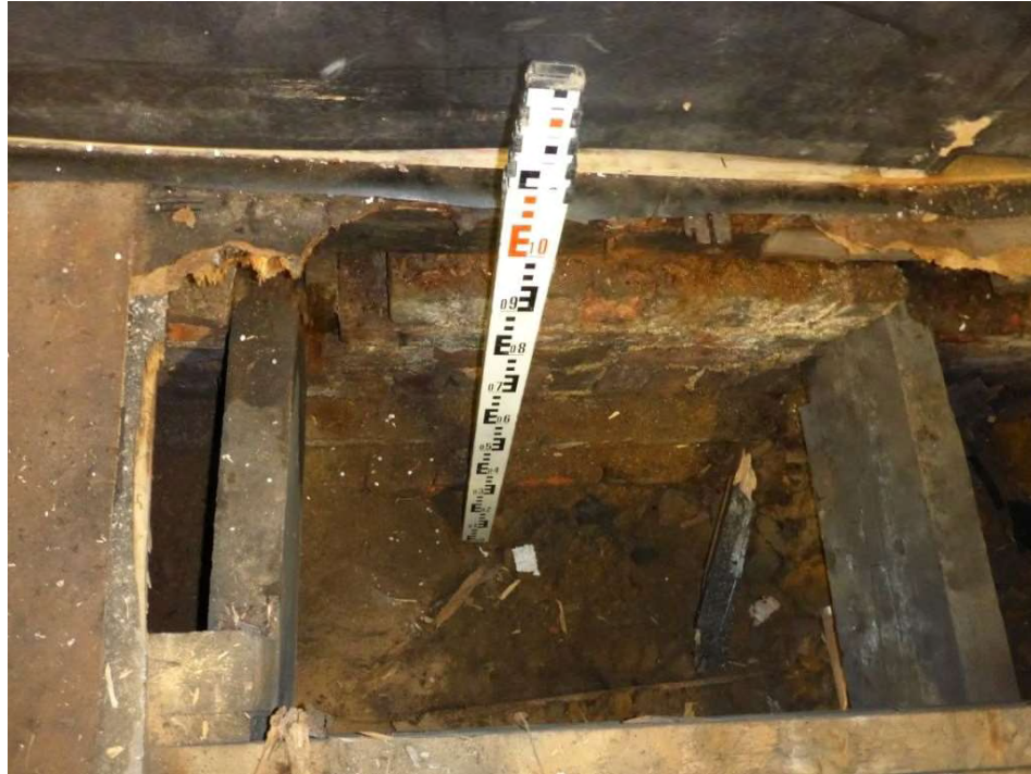
Trial Pit JTP06 - Photo 1
