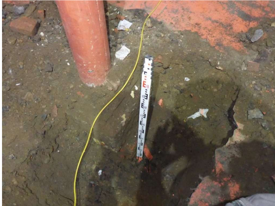
Trial Pit JTP01 - Photo 1
