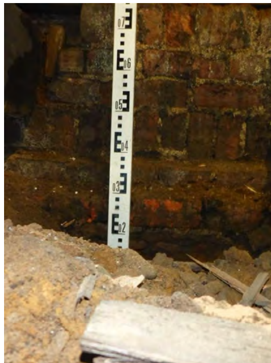
Trial Pit JTP06 - Photo 2
