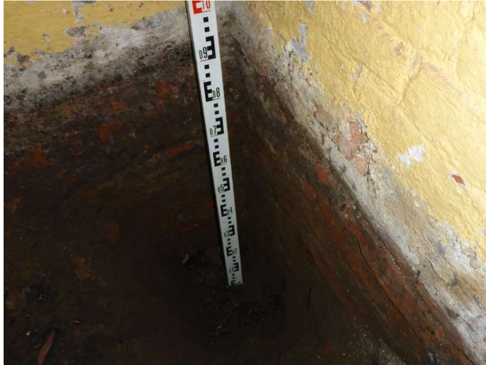
Trial Pit JTP03 - Photo 1
