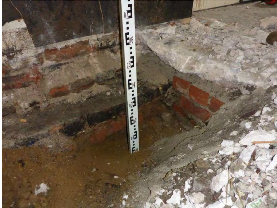
Trial Pit JTP05 - Photo 1
