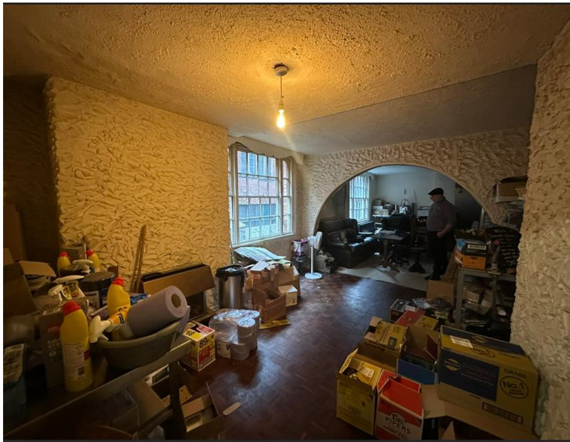
First floor – General view looking south-west across the southern rooms. The walls have been covered in thick plaster/ Artex and there is a late 20thC gas/electric fire installed. The floor is c.1960s/70s.
