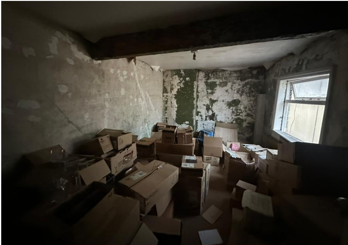
Second Floor – room to the north-west corner; the wall to the left bisects the historic fireplace/ chimney breast.
