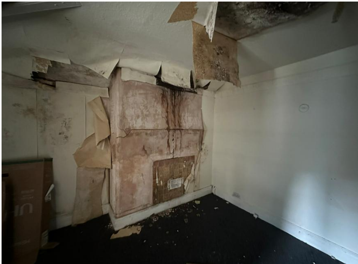
Second Floor – View looking south-west of the room to the south-eastern corner. The fireplace has been blocked.
