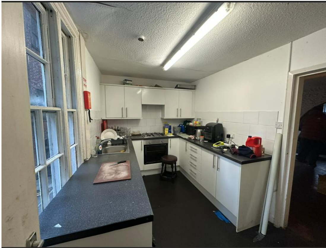
First floor – Room to the south-east corner which has been fitted out as a kitchen.
