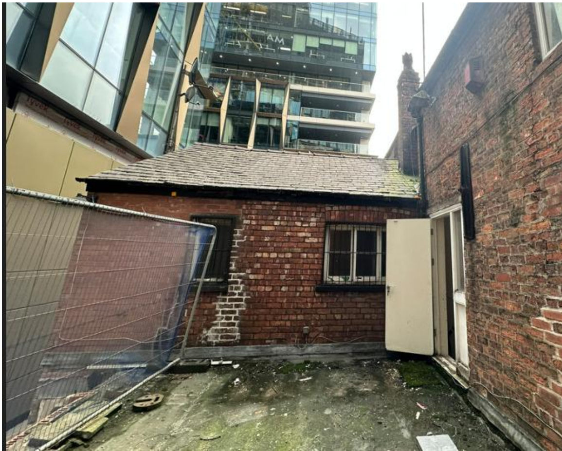
West elevation to first floor of eastern range illustrating areas of new brick to the left (north) end due to possible bomb damage
