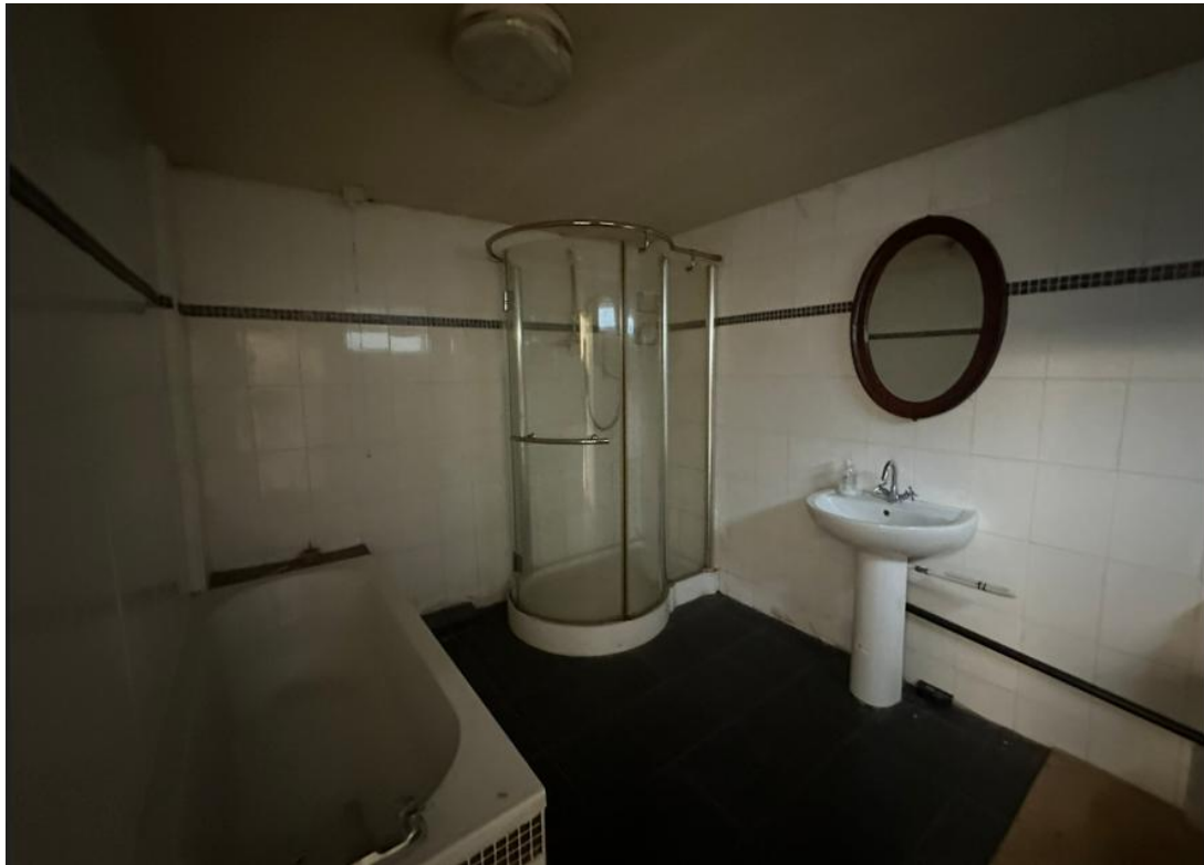
First Floor – View looking north-west of the room to the north east end of the building which has been converted into a bathroom.
